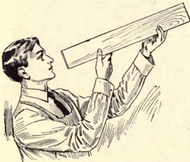
Fig. 32—Sighting for Straightness of Edge
