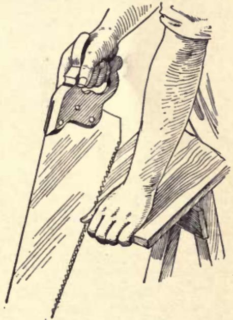
Fig. 14—Guiding the Saw with Left Thumb
