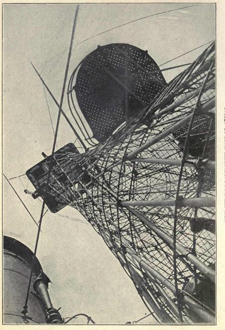
NEW STYLE OF BATTLESHIP MAST OR AËRIAL Showing Construction of the Type of Tower which now carries the Wireless. Photograph was taken from Base of Mast.
