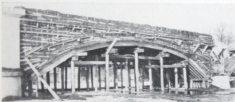
Bridge constructed in Waterloo, Iowa, during winter of 1921. No difficulty was experienced in this method of protection. Arch ring and hand rail are protected by the use of manure.
