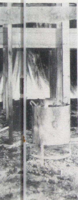
Workers under canvas and behind canvas placed concrete and maintain temperature.
