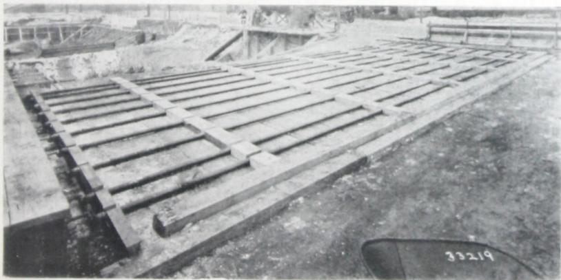
Special pipe grillage for heating aggregates installed by Thompson Starrett Co. The picture at the top of the page shows the complete installation of pipes, boiler and mixer. Note steam boiler has been removed from mixer frame and used to heat water in tank on top of mixer; electric motor substituted for former steam motive power. Loaded trucks of sand and gravel were dumped directly on to this platform. As soon as covered to a depth of 3 feet, steam is turned on continuously day and night. The lower picture shows a close-up of the arrangement of the pipe. Grillage drips for condensation are shown on the left hand side. This installation produced an aggregate with a temperature of approximately 70 degrees at all times.
