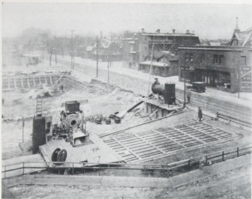
Special pipe grillage for heating aggregates installed by Thompson Starrett Co. The picture at the top of the page shows the complete installation of pipes, boiler and mixer. Note steam boiler has been removed from mixer frame and used to heat water in tank on top of mixer; electric motor substituted for former steam motive power. Loaded trucks of sand and gravel were dumped directly on to this platform. As soon as covered to a depth of 3 feet, steam is turned on continuously day and night. The lower picture shows a close-up of the arrangement of the pipe. Grillage drips for condensation are shown on the left hand side. This installation produced an aggregate with a temperature of approximately 70 degrees at all times.
