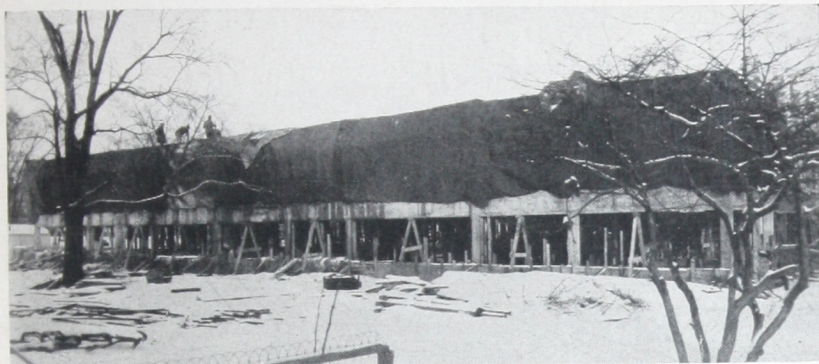
This 48-apartment building in Milwaukee was completed in time for spring occupancy because the work on the reinforced concrete structural frame was continued without interruption through January, 1923.
