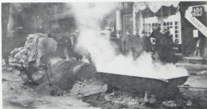
Method of heating water for concrete work shown in picture above.
