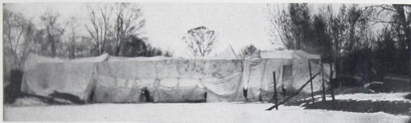
By being completely inclosed with canvas the concrete bridge over the Little Goose River in Sheridan County, Wyo., was completed during the severe cold weather of the winter of 1919 and 1920, and thereby permitted the opening of an important highway to spring traffic.
