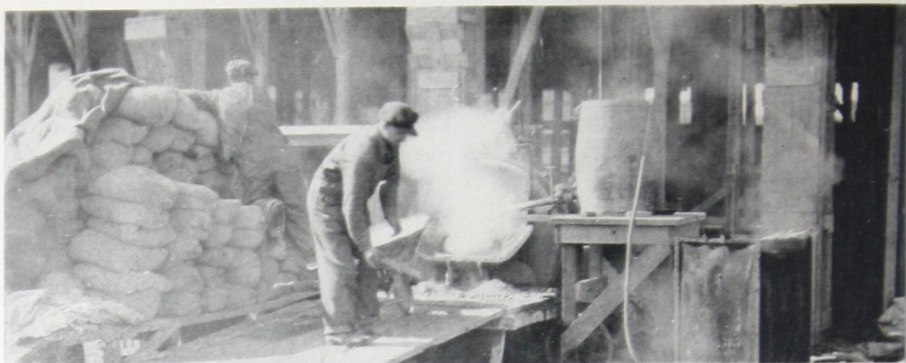
A Coke-burning hot water heater is very convenient for heating water close to the mixer.
