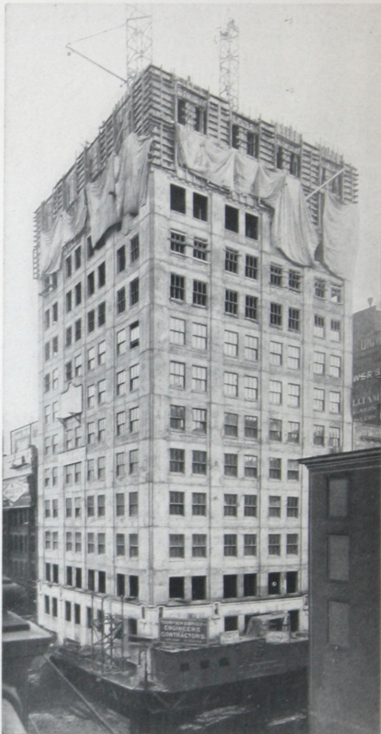
Cold weather need not delay the construction of tall concrete buildings. Construction of the 18-story Hide & Leather Building, New York, an all-concrete building, was carried on during the winter of 1920-21.
