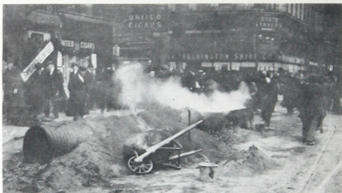
Repairing street car pavement at a busy corner in Chicago, sand and gravel being heated in a metal culvert and water in a flat tank.
