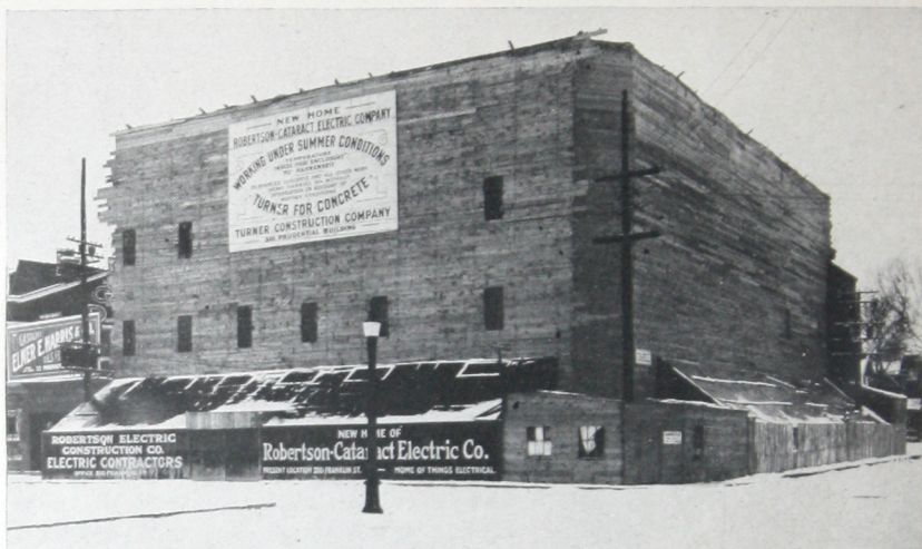
The Robertson-Cataract Electric Company's building in Buffalo was built in winter under summer temperature conditions. Complete inclosures, while costing more than temporary, movable ones, have the advantage of providing protection from the beginning to the completion of the work, for the workmen of all trades.
