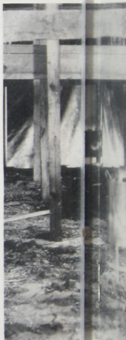
Salamanders under forms and be furnish heat for freshly placed co maintain constant temperature
