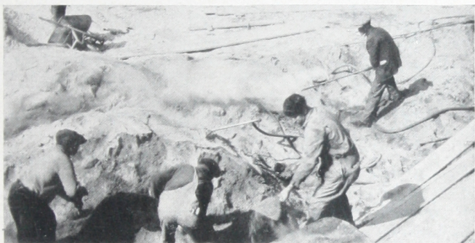
Steam jets placed in aggregate pile to keep the material from freezing. Frozen lumps may also be thawed out by the use of these jets.
