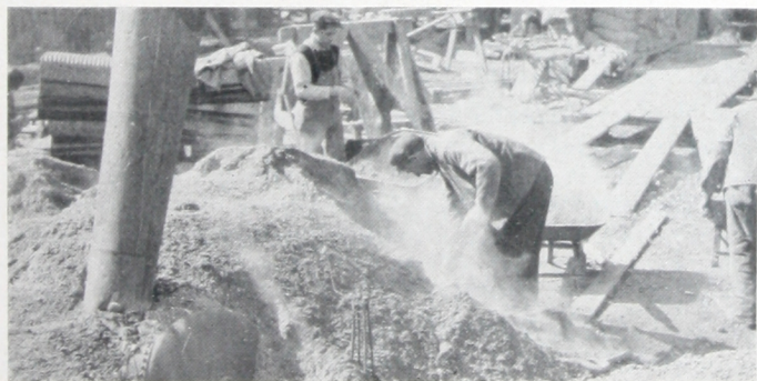
Another method of heating materials by the use of a coal fire in a discarded hot water boiler, seen in the lower left hand corner.
