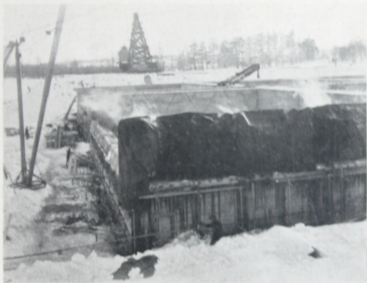
Winter concrete work on $3,000,000 sewage treatment plant at Worcester, Mass., during winter of 1922-1923.
