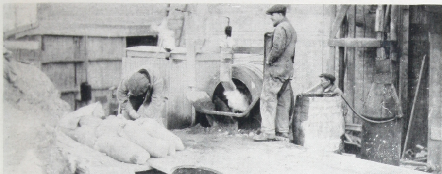
An oil-burning heater projected into the mouth of the mixer heats the materials sufficiently to keep the concrete from freezing, providing other precautions are used after placing in the forms.
