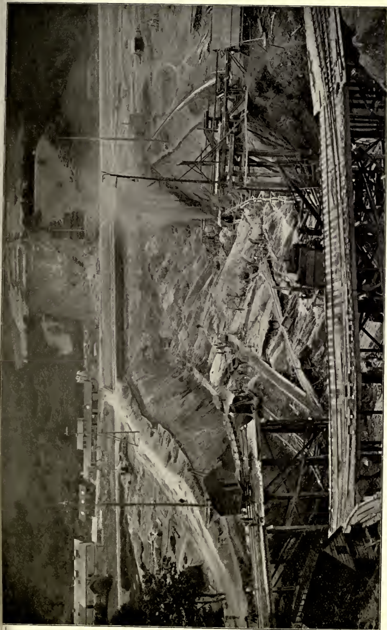
By permission of G. F. Deacon, C.E. No. 1. THE VYRNWY DAM—EXCAVATING THE TRENCH ACROSS THE VALLEY OF THE RIVER VYRNWY.
