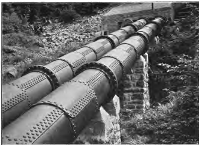
FIG. 45.—Riveted steel pipe lines for high pressure.
