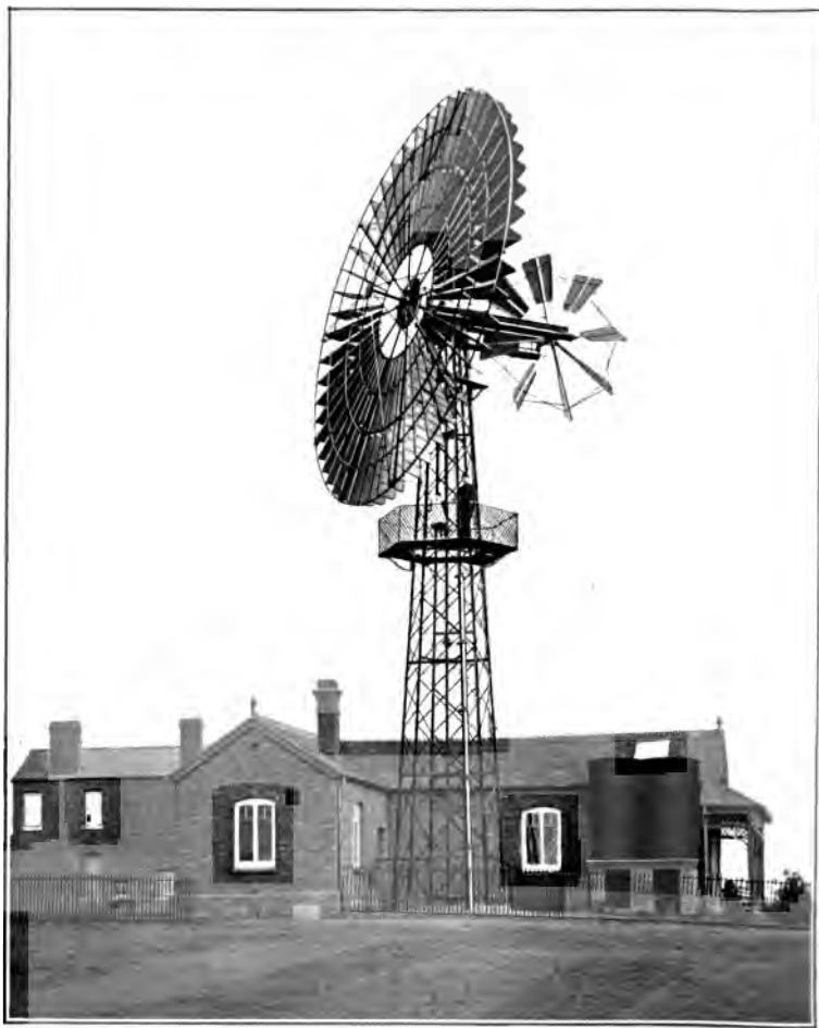
FIG. 103.—Windmill (35 ft. dia.) utilized for Pumping and Driving an Electric Generator.
