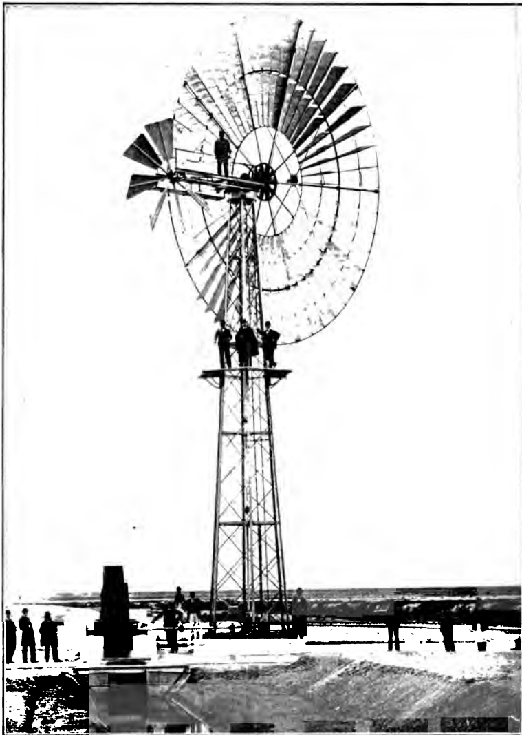
FIG. 82.—Windmill (37.5 ft. diam.) employed for Pumping.
