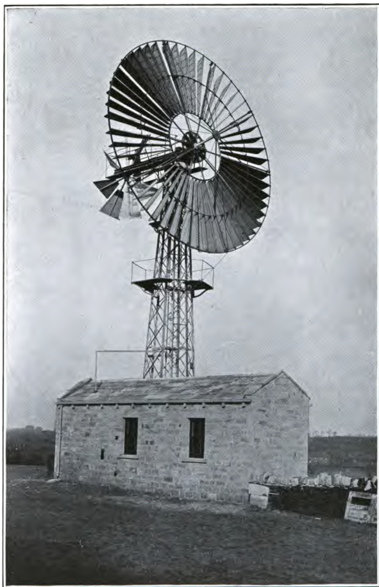
FIG. 81.—Windmill (30 ft. diam.) connected to Electric Generator.
