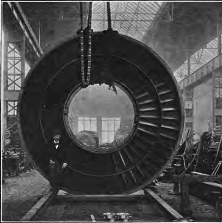
FIG. 43.—Jonval turbine working under a head of 2 feet.
