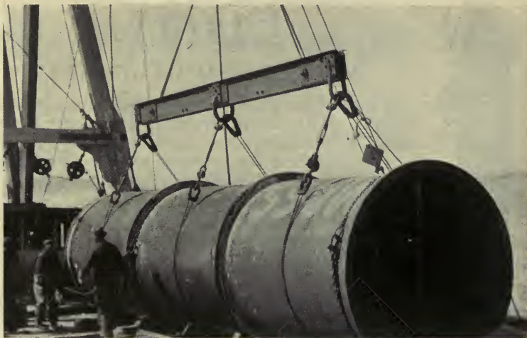
84" U. S. Cast Iron Pipe Outfall Sewer being installed by Metropolitan Sewer and Water Board, Boston, Mass.
