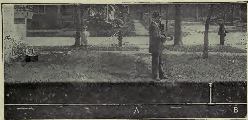
FIG. 284. — Manner of Using Wireless Pipe Locator.
