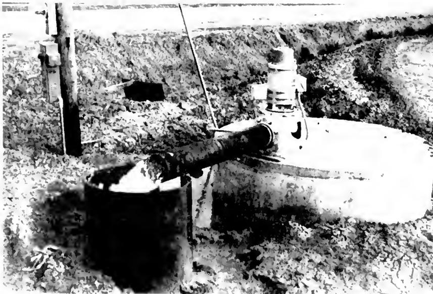
FIGURE 6. CONCRETE SUMP
