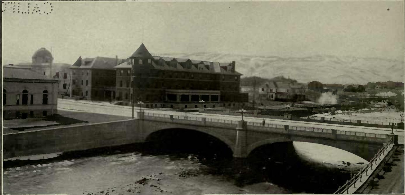
*The construction here necessitated a full consideration of the rapid current of the river and its heavy drift of ice in winter—seen in the illustration*
