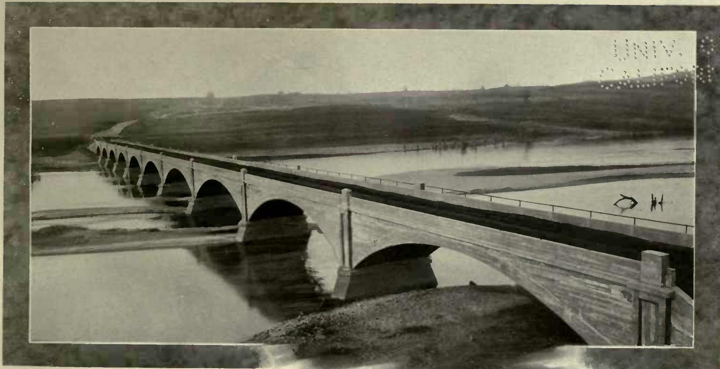
*Erected jointly by Fresno and Madera Counties. The simplicity of design of this massive structure, one of the largest in California, led to ease of construction and consequent economy*
