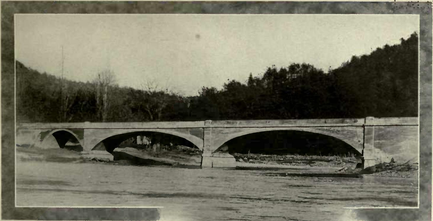
*Situated far up in the mountains, this structure is interesting because of the extreme depth excavated to reach bedrock, the bottom of the mid-river pier being nearly 30 feet below the water*
