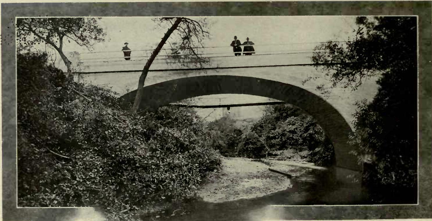
*The curve of this bridge is designed to afford ample passage for flood water, while conforming to the low street grade*
