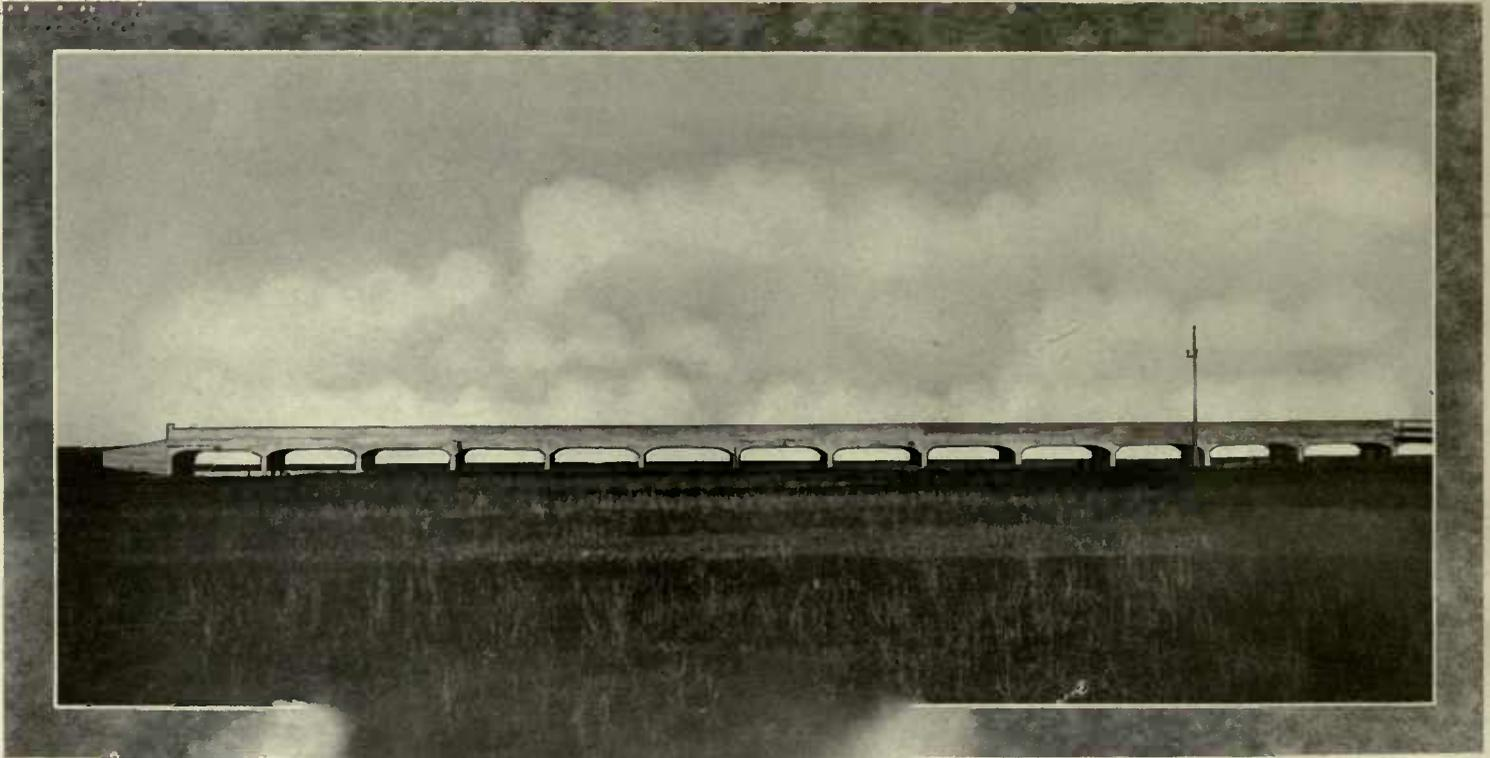
*This bridge has been built in sections of five spans at a time, and when completed will be 1100 feet long. Designed as a series of continuous flat spans, and remarkable for its low cost*
