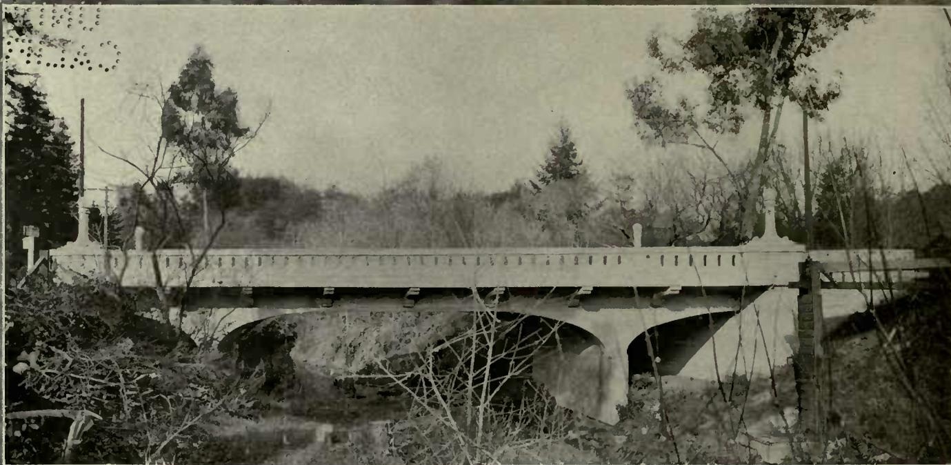
*Unique in being one of the first concrete bridges designed strictly on the cantilever principle, making possible a shallow depth in the carrying girders*
