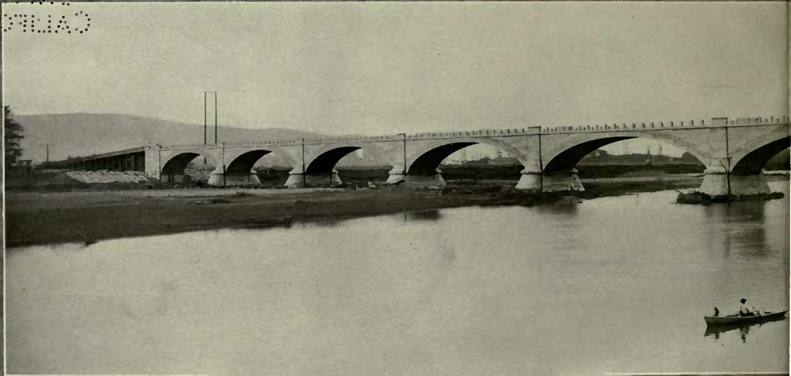
*One of the longest concrete bridges on the Pacific Coast. Each pier rests on 250 piles and is of extremely mass*
