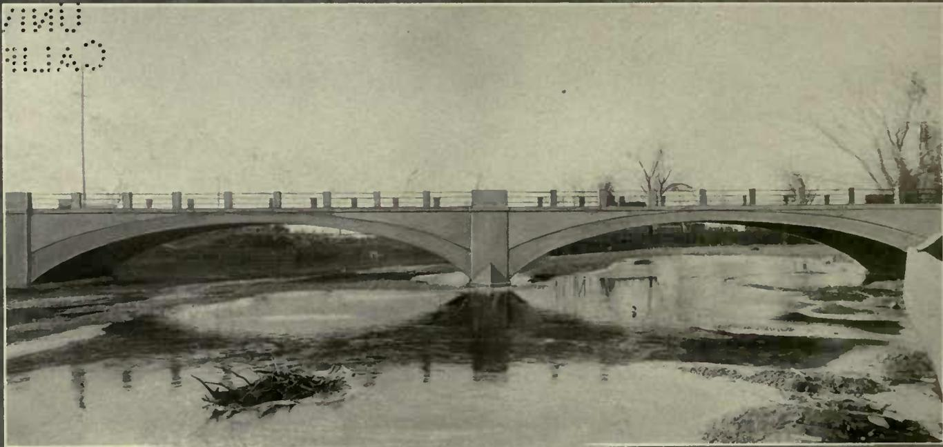
*Built to replace an old type combination structure of steel and wood. Notable for extremely low cost of construction*
