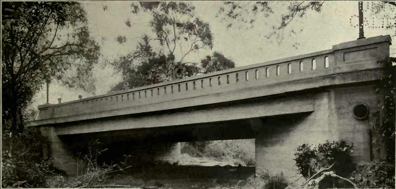
*An example of the concrete girder bridge, where a considerable rise of water between low banks was provided for*
