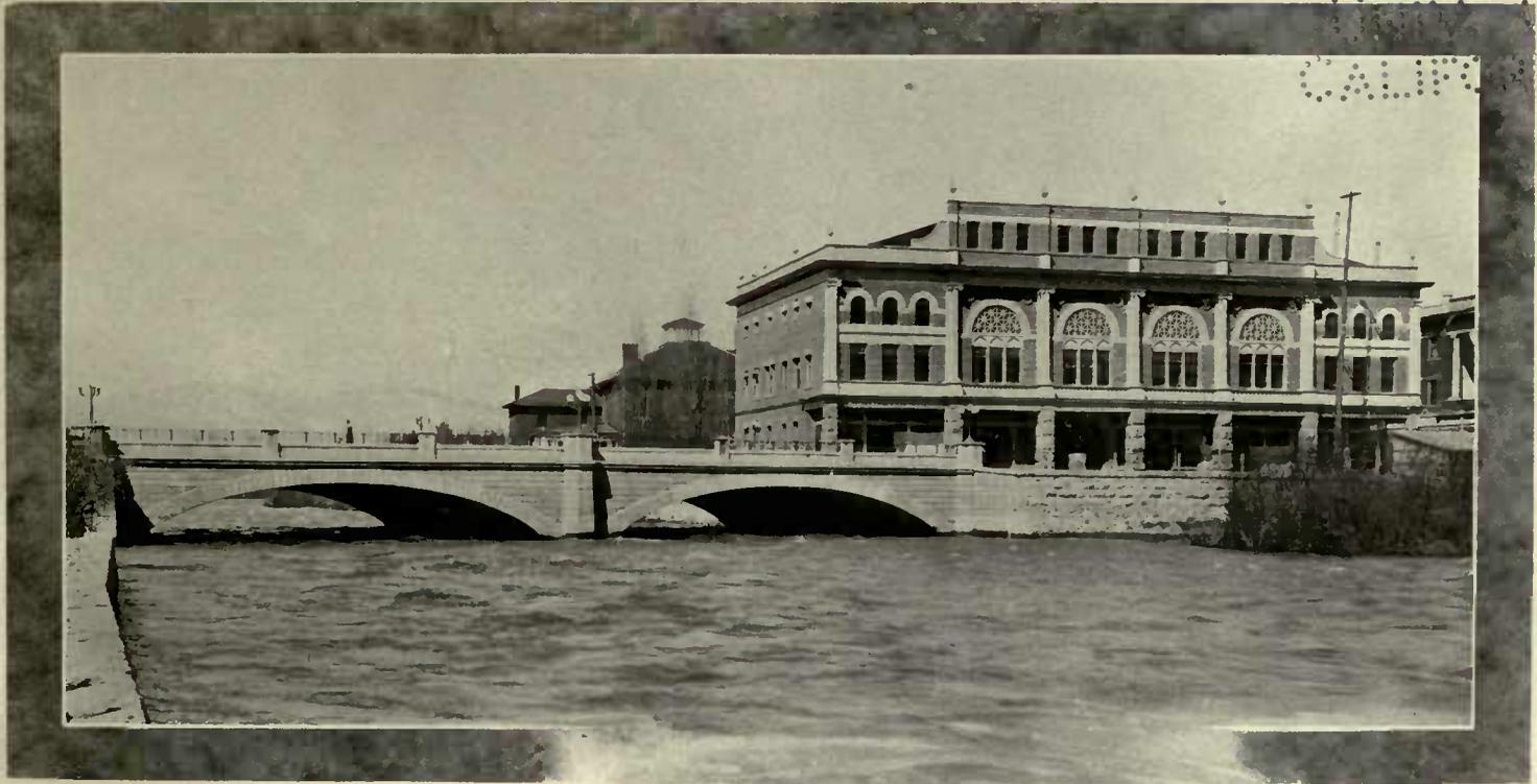
*This is one of the first bridges built on the Pacific Coast of reinforced concrete—a pioneer. The only bridge shown, not in California*
