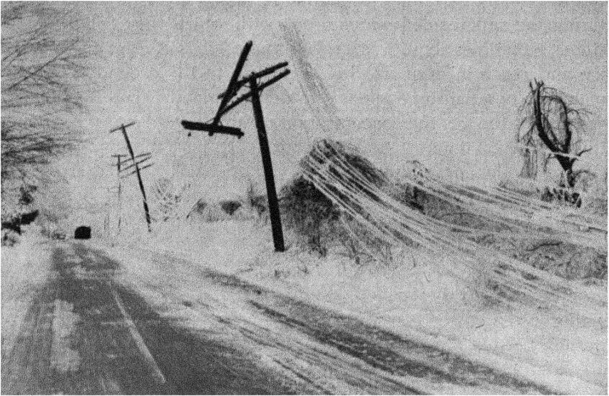
Fig. 67. Telephone Lines and Trees Broken by the Weight of Glaze Ice Near Mount Freedom, New Jersey, January, 1953. Damage to communication lines becomes severe when the diameter of ice covering the wires exceeds  $\frac{3}{4}$  inch. The Bell Telephone System suffered damages of \$8,000,000 from a single ice storm in January, 1951. *Courtesy, Southwestern Bell Telephone Company.*
