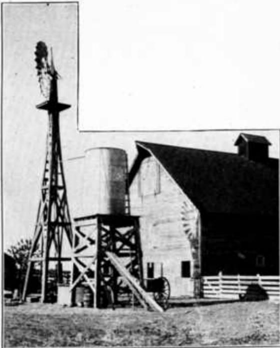
FIG. 42.—Galvanized-iron tank on timber trestle, Herington, Kans.
