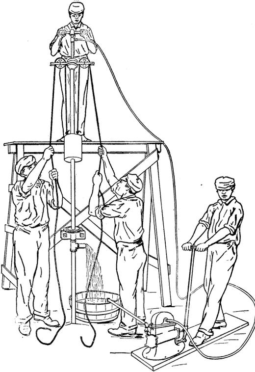
FIG. 25.—Driven well and application of the jetting process.
