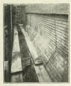
FIG. 6—SCRATCH COAT ON FLOW PARTITION.
