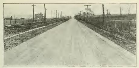
SECTION OF ELEVEN-MILE EXTENSION OF DIXIE HIGHWAY WITH KENTUCKY ROCK ASPHALT SURFACE AS DESCRIBED IN THIS ARTICLE.
