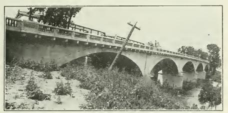
VIEW OF SIX SPAN REINFORCED CONCRETE HIGHWAY BRIDGE OVER WABASH RIVER AT ATTICA, IND.
