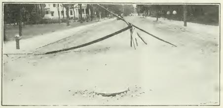
VIEW OF WATERBOUND MACADAM PAVEMENT IN STEVENS POINT, WIS., READY FOR RESURFACING WITH ASPHALTIC CONCRETE.
