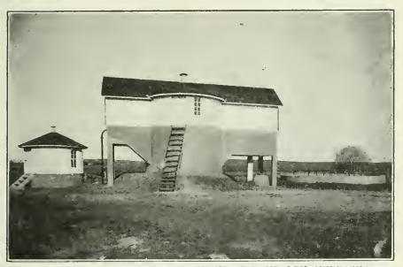
VIEW OF SEWAGE TREATMENT PLANT AT RANDOLPH, NEBRASKA. Pump Sump on Left, Settling Tank in Center and Sprinkling Filter Bed on the Right. A Sludge Bed Lies Directly Back of the Settling Tank.
