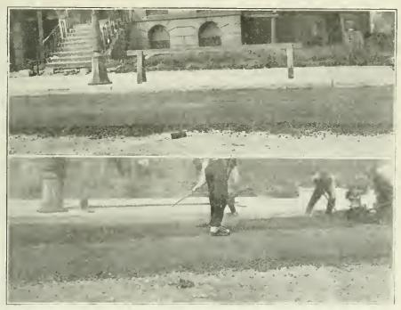
VIEWS SHOWING CONSTRUCTION OF ASPHALTIC CONCRETE BASE FOR SHEET ASPHALT PAVEMENT ON WASHINGTON BLVD., CHICAGO. Left: Macadam Foundation and First Layer of Black Base Partially Rolled. Right: Raking Second or Final Layer of Black Base.
