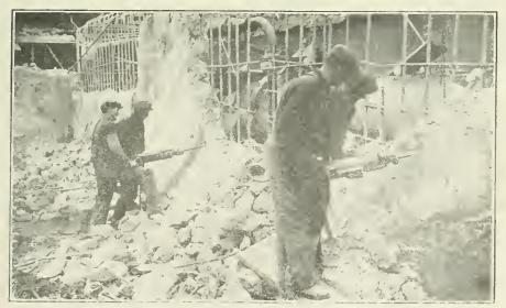
REMOVING REINFORCED CONCRETE VENTURI METER VAULT WITH COM-PRESSED AIR OPERATED "PAVING BREAKERS," AT WATER FILTRATION PLANT, CLEVELAND, OHIO.
