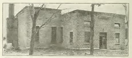
FIG. 1—ELECTRIC LIGHTING POWER PLANT AT ARCADE, N. Y.. DIRECTLY ACROSS STREET FROM SCHOOL BUILDINGS AND BLOCK FIRST HEATED BY EXHAUST STEAM FROM THIS 475 B. H. P. PLANT.
