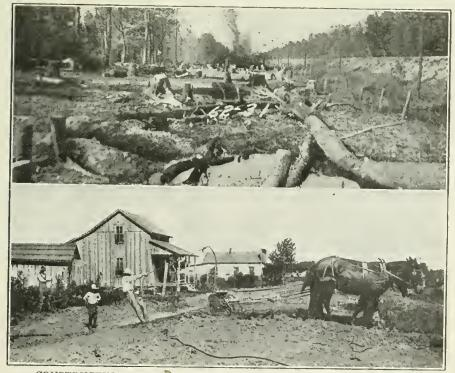
CONSTRUCTING OZARK TRAIL HIGHWAY IN EASTERN ARKANSAS. Clearing Heavy Growth of Timber from Right of Way, Blasting Stump in Background —Dressing Embankment with Fresno.
