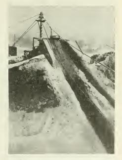
SHOWING INCLINE FROM GRAVEL PIT AND SAUERMAN SCRAPER DISCHARG-ING ITS LOAD THROUGH TRAP ONTO GRIZZLY.
