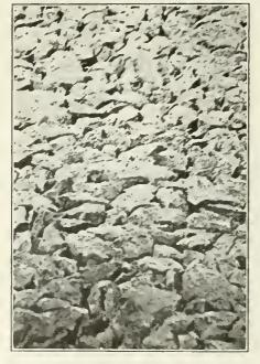
TYPICAL APPEARANCE OF TOP COURSE OF STONE SHOWING VOIDS LEFT OPEN TO GIVE ANCHORAGE FOR ROCK ASPHALT.
