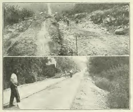
VIEWS ON CONSTRUCTION OF DANIELSON PIKE IN RHODE ISLAND. Views Show Typical Excavation and the Laying of Bituminous Concrete Pavement.
