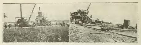
CONCRETING ON F. A. ROAD PROJECT NO. 43, MUSKEGON COUNTY, MICHIGAN. Left: Mixing Plant and Batch Handling Crane, Note Bottom Dump Batch Box. Right= Battery of Finishing Machines Following 2-yd. Paver.
