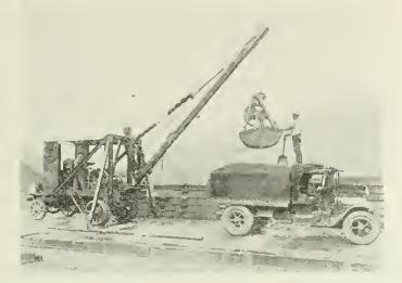
THE BYERS "TRUCKRANE," A MODIFICATION OF THE AUTO-CRANE ADAPTED FOR MOUNTING ON A MOTOR TRUCK.
