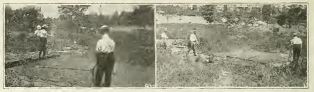
FIG. 5—VIEWS SHOWING SPRINKLING OF TEST PLOTS IN DETERMINING RELATION BETWEEN RAINFALL AND RUNOFF AT ST. LOUIS.
