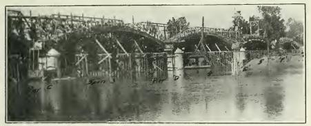
CENTERING IN POSITION TO POUR NORTH HALF OF ARCH, SPAN NO. 1, ATTICA, IND., HIGHWAY BRIDGE.
