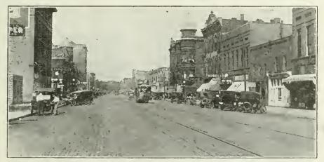
BRICK PAVEMENT WITH ASPHALT FILLER ON MAIN STREET, GALESBURG, ILLINOIS, AFTER SIX YEARS' SERVICE.
