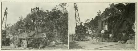
VIEWS OF HEAVY WATER PIPE LINE CONSTRUCTION AT NEW BEDFORD, MASS. Bucyrus Steam Shovel is Shown Dumping to Motor Truck Body Direct. Bucyrus Steam Crane Used in Handling Pipe and Other Purposes on the Job.
