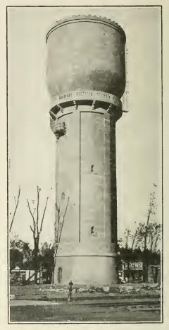
FIG. 1—REINFORCED CONCRETE WATER TOWER AND TANK AT BRAINERD, MINN.
