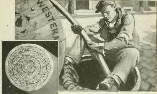
2400 telephone wires in a cable little larger than a man's wrist.
