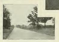
**TEXACO** Sheet Asphalt on Route 82. Work done by Smith Construction Company. (Blast furnace slag used in concrete foundation.)
