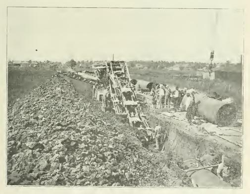
NO. O AUSTIN TRENCHER, WITH SUPPLEMENTARY WIDENER, DIGGING 4<sup>1</sup>/<sub>2</sub> MILES OF 7x7 FT, TRENCH FOR 48 IN, GAS MAIN FOR PEOPLES GAS LIGHT AND COKE CO. OF CHICAGO.
