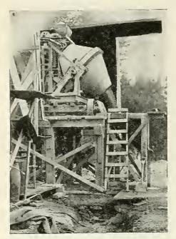
VIEW OF THE 10-S SMITH TILTING MIXER USED ON CONSTRUCTION OF THE NEW WATER RESERVOIR AT OMAHA, NEB, A POWER LOADER AND EXTENDED TRACK MAKES IT POSSIBLE TO TAKE AGGREGATE FROM LOWER LEVEL TO THE HOP-PER ABOVE.
