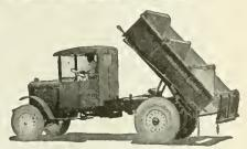
Kissel special Road-builder's Truck with body divided for three batches of one cubic yard each.
