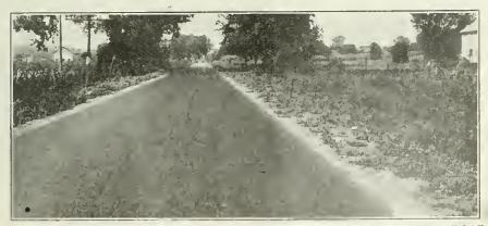
FIG. 1-BRICK PAVEMENT ON DAVENPORT-PRINCETON (IOWA) ROAD FOLLOWING THE MISSISSIPPI RIVER BETWEEN DAVENPORT AND CLINTON. SCOTT COUNTY (IOWA) HAS 23 ½ MILES OF THESE PAVEMENTS, BUILT AND BUILDING.
