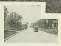
Texaco Sheet Asphalt on "F" Street, Lincoln, Nebraska. Laid 1916 -no maintenance to date.
