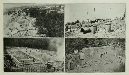
VIEWS ON CONSTRUCTION OF CAMP PIKE CANTONNENT. FIG. 1—PUMP HOUSE WITH PUMP INSTALLED AND WALLS BEING BUILT. FIG. 2—AIR COMPRESSOR PLANT AND ELECTRIC LIGHT AND POWER LINES ON 23-FOOT SEWER CUT. FIG. 3—SEPTIC TANK READY FOR ROOF. FIG. 4—NATIVE STONE ARCH FOR CARRYING SEWER ACROSS RAVINE.
