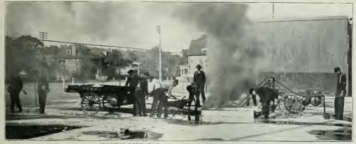
"PLUTO" PORTABLE ASPHALT HEATER ON THE JOB.
