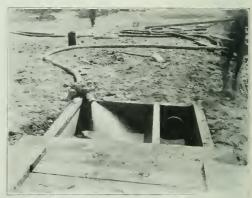
SETTLING BASIN, SHOWING POSITION OF OUTLET PIPE BACK TO SEWER.
