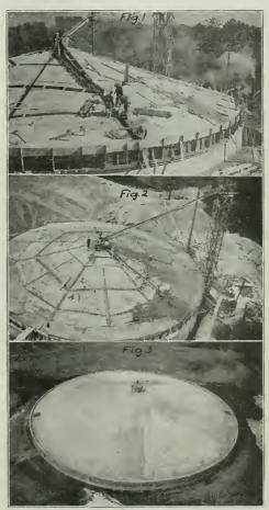
CONSTRUCTION VIEWS ON MANKATO RESERVOIR. FIG. 1—POURING THE ROOF BEAMS. FIG. 2—POURING THE ROOF, FIG. 3—ROOF JUST COMPLETED, GROUT SURFACE WASH NOT YET FINISHED.
