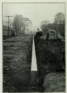
CURB MADE WITH WELL-ALIGNED, RIGIDLY-HELD FORMS.
