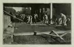
RELAYING OLD SAND FILLED BRICK PAVEMENT MONOLITHICALLY, CHAMPAIGN, ILL.
