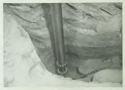
BOTTOM OF SUCTION PIPE ON THREE MILLION CENTRIFUGAL PUMP.
