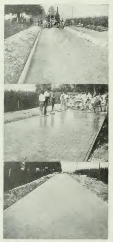
VIEWS SHOWING CONSTRUCTION OF WIRE-CUT LUG MONOLITHIC BRICK HIGHWAY, ED-GAR COUNTY, ILL.
