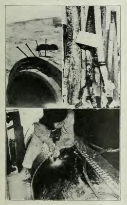
EFFECTS OF ELECTROLYTIC ACTION ON SEATTLE WATER PIPES. LOWER VIEW SHOWS MAIN BEING CUT FOR REPAIR.
