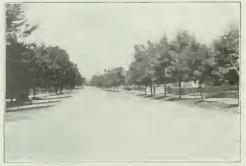
VIEW OF BITUMINOUS MACADAM ROAD BUILT BY PENETRATION METHOD, WAYNESBORO, VA.
