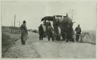
STANDARD METHOD OF APPLYING ASPIJALT MACADAM BY PENETRATION METHOD WITH PRESSURE DISTRIBUTOR WAGONS.
