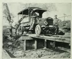
CALIFORNIA HIGHWAY COMMISSION'S ROAD-RE-PAIR GANG WITH MOTOR TRUCK CONSTRUCTING TEMPORARY BRIDGE OVER WASH-OUT IN A STATE ROAD.
