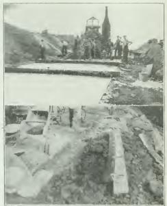
PLACING EXPANSION JOINTS IN BALTIMORE ROAD, LOWER VIEW SHOWS HOW JOINT IS CLAMPED TO BRIDGE
