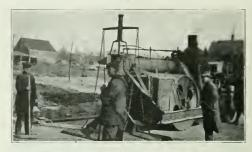
MELTING SNOW FROM UNFINISHED PAVEMENT WITH ASPHALT ROAD HEATER.
