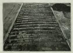
ALTERNATE ROWS OF WOOD AND BRICK IN TRACKS OF TOLEDO RAILWAYS & LIGHT CO., TOLEDO, OHIO.
