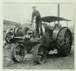
OIL TRACTOR RIGGED WITH POWERFUL HOIST
