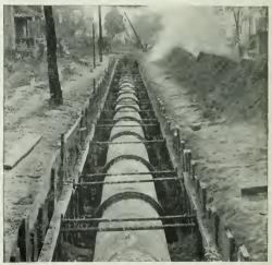
EXTENSIBLE BRACES IN PLACE IN A TRENCH EXCAVATION.
