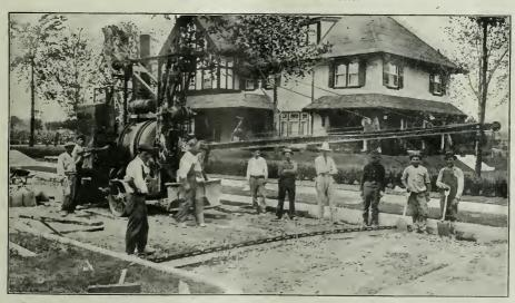
McKINLEY PLACE, GRÖSSE POINT, MICH. MASON L. BROWN, ENGINEER; MYERS & LABADIE, CONTRACTORS. A TWO-COURSE CONCRETE PAVEMENT, SHOWING TRUS-CON ARMOR PLATES IN POSITION READY FOR CONCRETE. THESE HAVE BEEN PROPERLY PLACED WITH THE TRUS-CON INSTALLING DEVICE, WHICH ASSTRES ARSOLUTE ACCURACY
