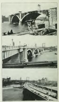
VIEWS OF THIRD AVENUE, SOUTH, CONCRETE-STEEL ARCH BRIDGE, MINNEAPOLIS, MINN. UPPER— SPANS 8 AND 9 SHOWING TRANSVERSE WALL FORMS AND FLOOR SLAB FORMS. MIDDLE—PERSPECTIVE VIEW SHOWING LAMP POLES, BRACKETS AND TWIN CABLEWAY TOWERS. CLEAR SPAN OF CABLEWAYS 2,036 FT.; MAX. LOAD PER CABLE 10 TONS; WORKING LOADS 6 TONS. LOWER—TOP VIEW OF STRUCTURE SHOWING CURVATURE ALIGNMENT.
