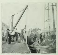
CONTRACTOR'S IMPROVED EQUIPMENT FOR DRIVING SHEET PILING.
