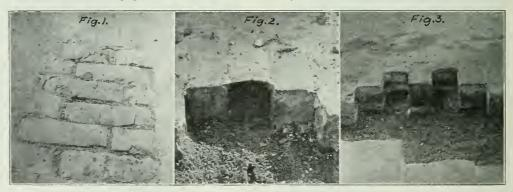
VIEWS SHOWING FAILURE OF BRICK PAVEMENT DUE TO IMPERFECT GROUTING FIG. 1—DEFECTIVE SPOT BEFORE OPENING. FIGS, 2 AND 3—VIEWS FROM OPPOSITE SIDES OF OPENING.
