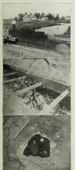
VIEWS SHOWING FEATURES IN UNDERGROUND CONSTRUCTION: 1—LIGHT WEIGHT CORRUGATED SHEET STEEL PHANG AS USED IN TRENCH WORK; 2—TRIPOD'DRILLS IN DES PERES (ST. LOUIS) FOUL WATER SEWER; 3—MEETING OF HEADINGS IN HUDSON RIVER SIPHON TUNNEL. POINT SHOWN IS BENEATH RIVER NEAR WEST POINT, N. Y.
