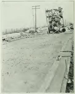
VIEW SHOWING CASTING CONCRETE CURB INTEGRAL WITH BASE, MONROE-TOLEDO ROAD CONSTRUCTION.
