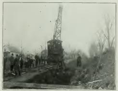
FIG. 2 LOCOMOTIVE CRANE WITH ORANGE PEEL BUCKET IN SEWER EXCAVATION.
