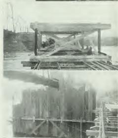
VIEWS SHOWING COFFERDAM FRAME AND SHEET STEEL PILE TENPLATE AND PILING.
