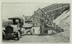
MECHANICAL LOADER CARRYING GRAVEL DIRECT FROM PILE TO TRUCK.
