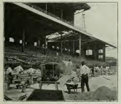
VIEW SHOWING LAYOUT OF CONCRETING PLANT USED IN ENLARGING SEATING CAPACITY OF WHITE SOX BALL PARK BEFORE WORLD'S SERIES.
