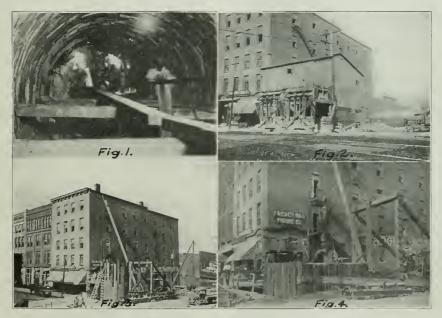
CONSTRUCTION VIEWS ON MILWAUKEE SEWER SIPHON TUNNEL UNDER RIVER. FIG. 1—HITTING DAYLIGHT—SHIELD JUST EMERGING AT RISER SHAFT—NOTE KEYBOARD AND TIMBERING. FIG. 2—HOUSING OVER DROP SHAFT. FIGS. 3 AND 4—METHOD OF DRIVING INNER SET OF 50-FT. BY 14-IN. LACKAWANNA STEEL PILING AT DROP SHAFT.
