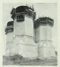
EASTERN HILLS STANDPIPES, CINCINNATI WATER WORKS, ENCASED IN ORNAMENTAL CONCRETE SHELL.
