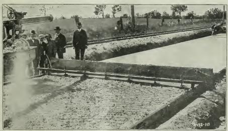
KAHN ARMOR PLATE FOR JOINT PROTECTION, SHOWING SPACES BETWEEN T-RAIL DEVICE AND PLATE WHICH ALLOWS PAVEMENT TO BE FINISHED FLUSH WITH TOP OF JOINT. KAHN ROAD MESH USED AS REINFORCEMENT.
