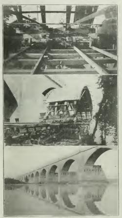
VIEWS OF CONCRETE ARCH VIADUCT ACROSS THE SUSQUEHANNA RIVER. 1—TRUCK RIGS FOR MOVING CENTERS: 2—CENTER READY FOR MOVING; 3—FINISHED ARCHES
