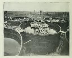
RAISING CONCRETE FORMS FROM FLOATS IN EN-CASING CINCINNATI STANDPIPES.
