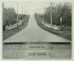
ILLUSTRATING COMBINATION OF ROAD MAKING MA-TÉRIALS TO WITHSTAND HEAVY HAULAGE.
