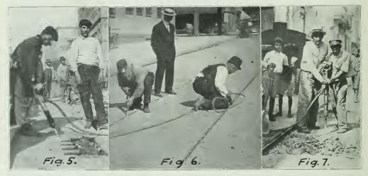
VIEWS ILLUSTRATING COMPRESSED AIR DRIVEN TOOLS ON STREET WORK. FIG. 5-REMOVING AND TOOTHING OUT BLOCK PAVING. FIG. 6-CUTTING ASPHALT WITH PNEUMATIC PAVEMENT PICKS. FIG. 7-ANOTHER CONCRETE CUTTING TOOL, THE PNEUMATIC TIE TAMPER, AT WORK.
