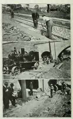
FIG. 3—SULLIVAN HAMMER DRILLS CUTTING AS-PHALT BLOCK PAVEMENTS AND CONCRETE BASE. FIG. 4—CHICAGO COMPRESSOR SUPPLYING PNEUMAT-IC RAMMERS IN TRENCH. FIG. 5—INGERSOLL-RAND PNEUMATIC TAMPING MACHINE RAMMING BACKFILL IN TRENCH.
