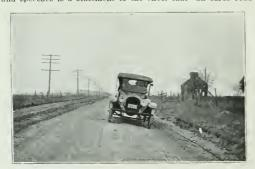
A SECTION OF THE DINIE HIGHWAY IN ILLINOIS. MISTREATED PERIODICALLY WITH A TRACTOR AND LEVELER. CROWN 2 1-5 IN. TO THE FOOT. UNCOMFORTABLE WHEN DRY—DANGEROUS WHEN WET.
