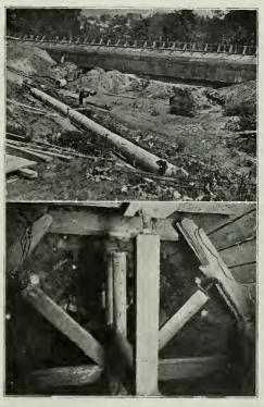
UPPER—VIEW OF 8-FT. AND 3-FT. CONCRETE SEW-ERS, TORONTO. LOWER—NEEDLE BEAM METHOD OF SUPPORTING SHEETING IN TUNNEL SECTION.
