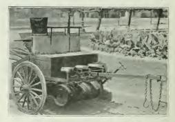
NEW HEATING FURNACE FOR BITUMINOUS PAVEMENT TOOLS.
