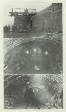
CONSTRUCTION VIEWS OF MILWAUKEE SEWER SIPHON TUNNEL. MIXER AND HOPPER AT TOP OF RISER SHAFT—OPERATING SHIELD IN TUNNEL—SECTION OF ARCH JUST INSIDE OF AIR LOCK.
