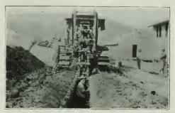
VIEW OF DITCHER CUTTING 1,300 FEET OF 5-FOOT TRENCH IN TEN HOURS.
