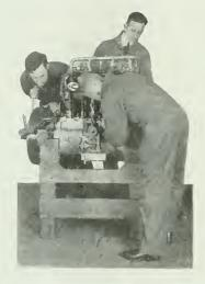
ASSEMBLING 2-TON TRUCK MOTOR; AT LEFT, TIMING ENGINE; AT RIGHT, FITTING WATER PUMP; IN FRONT, MOUNTING CARBURETOR.
