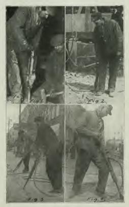
VIEWS ILLUSTRATING USE OF COMPRESSED AIR DRIVEN TOOLS ON STREET WORK. FIG. 1-BREAKING CONCRETE WITH JACKHAMER AND POINTED CHISEL BIT. FIG. 2-TEARING UP CONCRETE PAVING WITH PNEUMATIC RIVETER AND CHISEL. FIG. 3-CUTTING ASPHALT PAVING. FIG. 4-SCORING ASPHALT PAVING.
