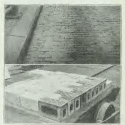
VIEW SHOWING WEAR OF BLOCKS ON BROOKLYN BRIDGE APPROACH. METHOD OF LAYING THE CE-MENT IRON BLOCKS. THESE BLOCKS GO NEXT TO CURB.
