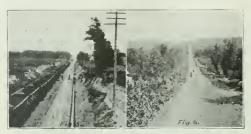
FIGS. 5 AND 6—SIXTEEN-INCH REDWOOD FORCE MAIN CONSTRUCTION BELOW AND ABOVE BOOSTER STATION.
