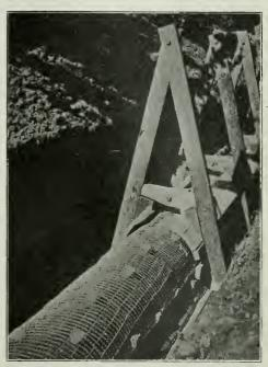
VIEW OF FORMS AND REINFORCING USED IN CONCRETE COVERING AN OLD STEEL WATER PIPE.
