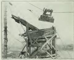
SLACK CABLE WAY EXCAVATOR WITH 31/2 FEET. CLEARANCE READY TO DUMP LOAD.
