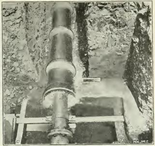
FIG. 3. METHOD OF INSULATING steam pipes laid in the street.
