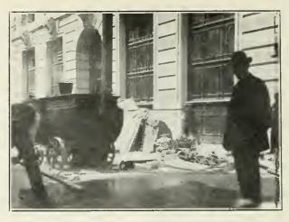
S QUEEGEEING the pitch flush coat applied to the surface of the blocks.
