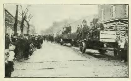
Wilmington, Del. Last of four 32-ton girders hauled on a 6-ton truck by 35 horses, November 28, 1911, over Bitulithic paving four years old at Fifth and Spruce Streets. These tremendous loads made not the slightest mark on the Bitulithic Pavement.
