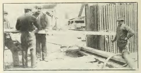
M ETHOD OF DRIVING sheet steel piling with water jet and the lever, chain and pawl shown.
