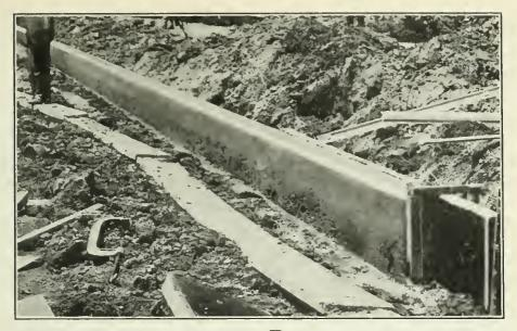
and steel forms are shown in place with the stakes for holding them rigid, the joint plates and the clamp for keeping the forms in exact position with respect to each other. Farther in the rear the concrete has been filled into the form and the first workman seen removes the joint plates and is seen placing the curb bar, which he does by forcing it into the wet
