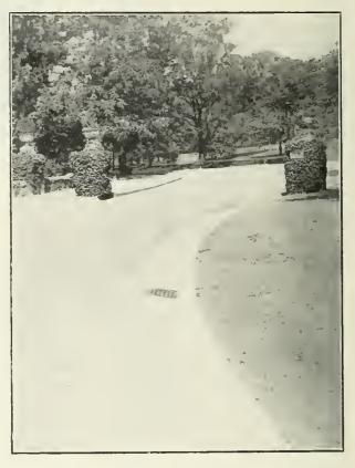
R EINFORCED CONCRETE INLET to sewer, showing its adaptability to concrete gutter on curve and without breaking the continuity of the concrete curbing.
