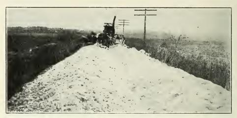
G RAVEL AND WASHED SAND aggregates deposited on the grade for feeding the concrete mixer shown in the background, on the Ellerton grade, near Bloomfield, Ind. Photographed by Engineer of Universal Portland Cement Company.
