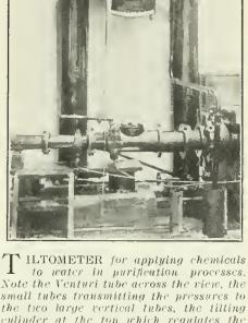
small tubes transmitting the pressures to the two large vertical tubes, the tilting cylinder at the top which regulates the flow of the chemical, and the funnel and tube which transmit the fluid to the water to be treated.
