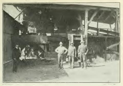
T HE WILMINGTON PAVING GANG on Twenty-second street, laying material. The wayon is just dumping a load of the bitulithic mixture on the shoveling boards.
