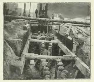
T RENCH for east line of piers on Franklin building, showing driving of foundation piles and use of sheet piling in excavating trench for concrete piers and walls.
