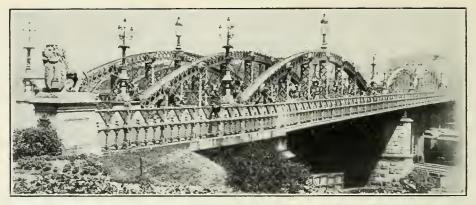
C ALVERT STREET BRIDGE over railroad and creek. A steel bridge, where girders beneath the floor were always in serious danger of corrosion by locomotive smoke.
