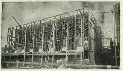
View of Cage containing 120 steel cells at the Hartford County Jail, Hartford, Conn. Erected by us before carrying up outside masonry walls.
