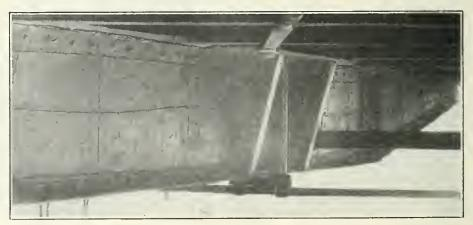
paint was removed, and the steel surface carefully exposed. Wire mesh reinforcement was earried all around the beams, held as shown in Sketch No. 1, and a coat of "gunite," 1½ inches in thickness, was applied; the gunite following the contour of these beams.
