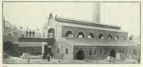
T HE REFUSE of the city of Northampton, England, is incinerated in this hightemperature plant, enlering from the left over the bridge, passing thru the furnace cells and removed as clinker on the floor below. A tall stack, shown in part, produces strong draft.
