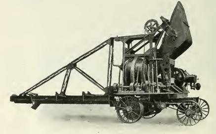
T HE MARSH-CAPRON CONCRETE PAVING MIXER. Note loading device and mixing delivery chute, which can discharge concrete at four points four feet apart.
