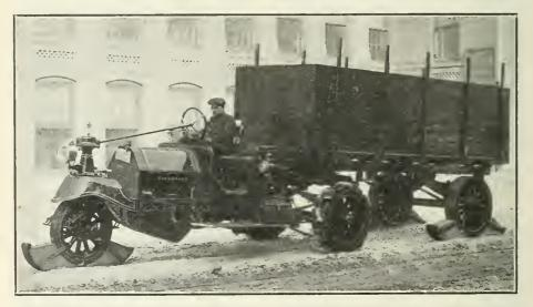
A NAUTOMOBILE on runners which is successfully used in a northern city having much snow.
