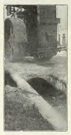
PART CIRCLE American ingot iron culvert, thirty-inch base, tcn-inch rise. Note heavy traction road machine carried by culvert.
