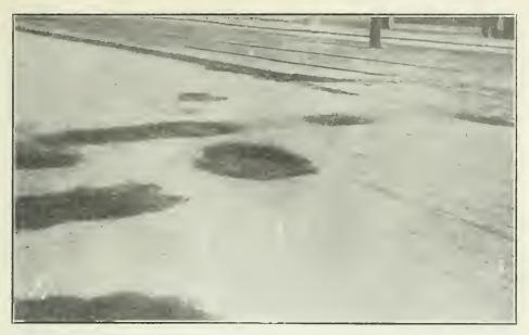
PORTION of Huntington Avenue, Boston, laid with broken stone treated with asphaltic materials applied by the penetration method, after four years of wear.
