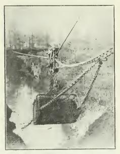
FIG. 1. Drag-line bucket excavator filled and emerging from wet gravel pit.
