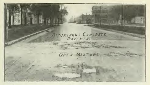
COMMONWEALTH AVENUE, Boston. Mass., showing contiguous sections of bituminous concrete and bituminous macadam laid in 1912 and their condition after about a year of use.
