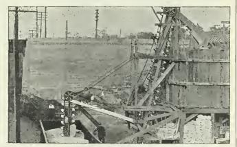
STATIONARY TYPE LINK-BELT CAR UNLOADER With two men trimming to the foot of the bucket elevator in the car,
