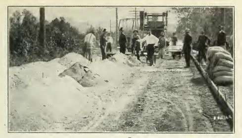
and gravel that was later used in the construction of the concrete pavement. The portion first built was good, while the other part was very defective. The cause of the difference, evidently, was due to the dirt and manure that had become mixed with the aggregates.
