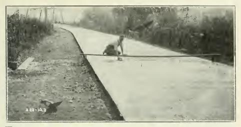
F INISHING THE SURFACE of a conerete pavement in Miami County, Ohio, with wooden float. Gravel shoulders will be placed along the side, Trussed Concrete Steel Company's joint protection.
