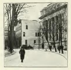
T HE completed granite block pavement with grout surface is as smooth as asphalt. The court house on the right makes less complaint of the noise, which was quite unbearable with the old pavement.
