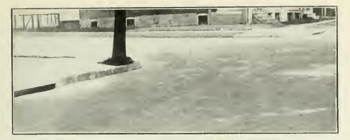
been designed and used in localities where it has been found necessary to place a great number of inlets to intercept surface water. These have been substituted where the use of so many iron inlet frames would have a tendency to disfigure and mar the curbing and general effect. It was found that this type of inlet was readily adaptable to all kinds of curves, without affecting their continuity.
