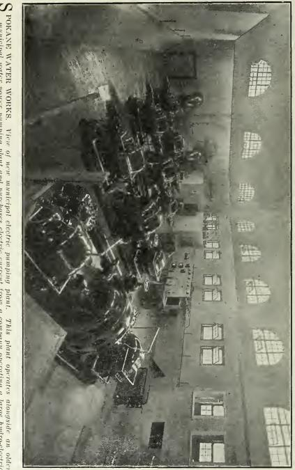
**S** POKANE WATER WORKS. View of new municipal electric pumping plant. This plant operates alongside an older municipal water power pumping plant and purchases electric current from a company operating a large hydro-electric power plant.
