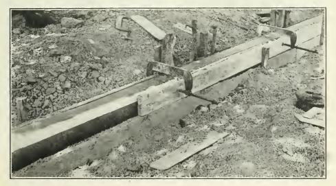
laid on Bewick Ave., St. Clair Heights, Mich., using wooden forms. Part of the form has been removed, showing part of the face as well as the top of the curh and the Trus-Con Curb Bar No. 1, which gives the rounded appearance to the curb corner.
