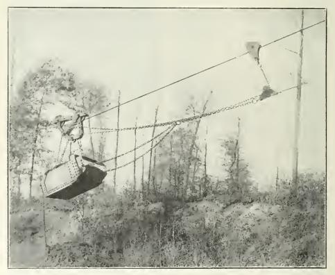
FIG. 2. Drag-line excavator bucket on its way from gravel pit to dump, side view. February, 1914
