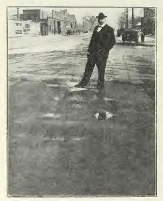
MASSACHUSETTS AVENUE, Cambridge, Mass. Section laid in 1908 with bituminous macadam by penetration method. Resurfaced three times and now in bad condition, as shown by photograph.
