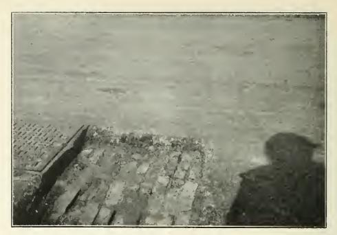
N INTH STREET, Wilmington, showing bitulithic laid on old brick pavement and a section taken up, to show high quality of the pavement thus made.
