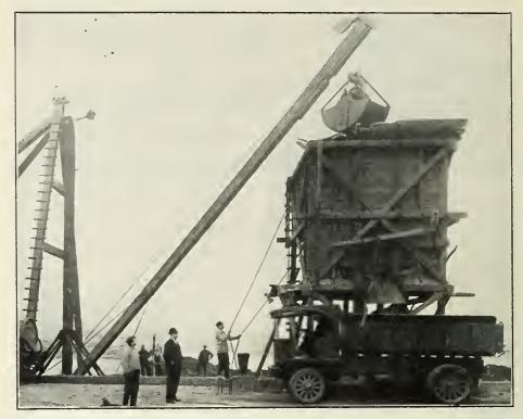
MOTOR TRUCK receiving broken stone from bin.on dock which is filled from the barge below by means of the bucket and crane.
