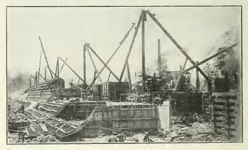
S TEVENS CREEK DAM under construction, as it appeared August 29, 1913. A completed portion of the spillway of the dam is seen in the background and the various sections in which the concrete was placed are shown by the work going on in the foreground.
