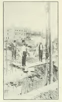
P ULLING STEEL SHEET PILING is simple with a gin pole and a small engine.
