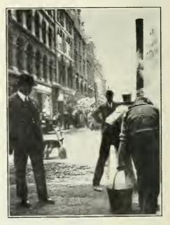
A PPLYING pitch coat to blocks. In the background the pitch coat has been followed by a flush coat of cement grout.
