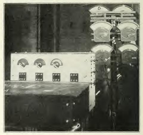
Plate No. 3 shows the operator's desk at the power station where voltage readings are taken. The regulating points are determined by the voltage setter from the indications of portable charts set at various points on the system, and those points are selected as the regulating points which give the best average results at the consumers' cut-outs.
