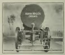
A NEW ROAD OILING MACHINE. Rear View Showing Control Mechanism.
