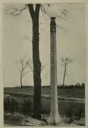
A Sample Post Showing Method of Inserting Street Signs by means of employing Bronze Letters set in the concrete.
