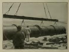
HANDLING 48-FOOT SECTIONS OF OUT-LET PIPE SUBMERGED IN BAY, NEW BEDFORD, MASS.
