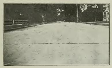
CONCRETE STREET IN FOND DU LAC, WIS. Transverse Joint, Showing Wear.
