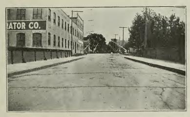
CONCRETE STREET IN FOND DU LAC, WIS. Note Transverse Joints and Longitudinal Cracks.
