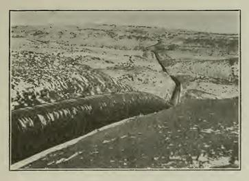
3. CONTINUOUS WOOD STAVE PIPE INVERTED SIPHON. Near Basin, Wyo.
