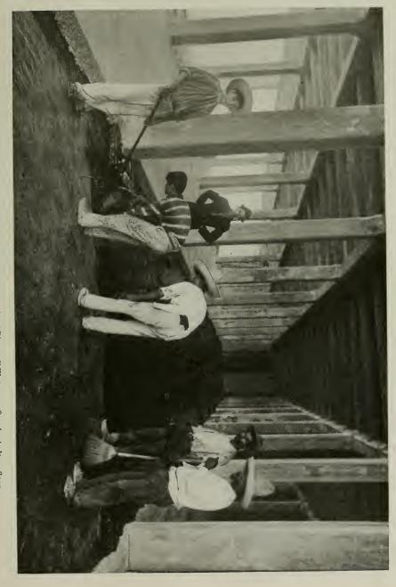
OBISPADO RESERVOIR, MONTERREY, MEX.-Laying "Pioneer" Waterproofing Asphalt on floor.
