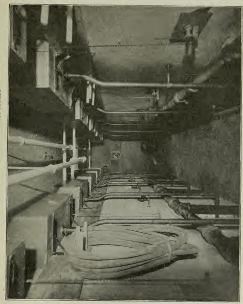
PUBLIC COMFORT STATION, BROOKLINE, MASS. III. Pipe-Chamber, Showing Piping for Water Supply.
