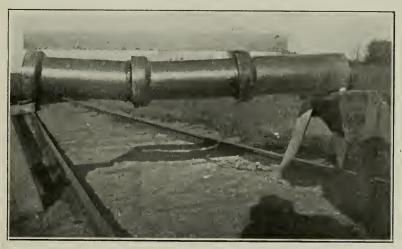
TEST OF G. K. WATER TIGHT SEWER JOINT.
