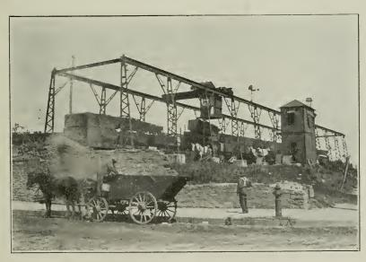
APPARATUS FOR TRANSFERRING GARBAGE WAGON BOXES TO CARS AT TRANSFER STATION, MINNEAPOLIS, MINN.
