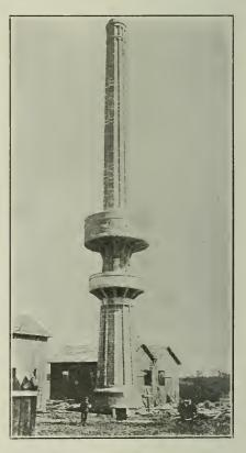
CONCRETE BLOCK CHIMNEY WITH TWO TWO REINFORCED CONCRETE RESERVOIRS
