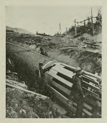
WOODEN STAVE PIPE LINE IN PROCESS OF CONSTRUCTION.
