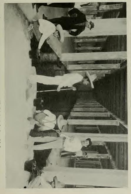
OBISPADO RESERVOIR, MONTERREY, MEX.-Painting the first layer of the floor.
