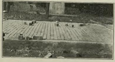
4. WIRE-CUT LUG BRICK PAVEMENT READY FOR FILLER.
