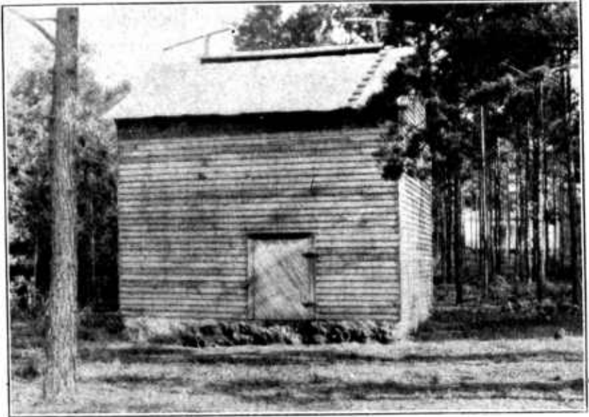
FIG. 2.—A 20 by 20 foot tobacco barn in North Carolina which was used for curing tobacco in 1921 during July and August and for sweet-potato storage in the autumn. The 8-inch tiles in the foundation provide floor ventilation.
