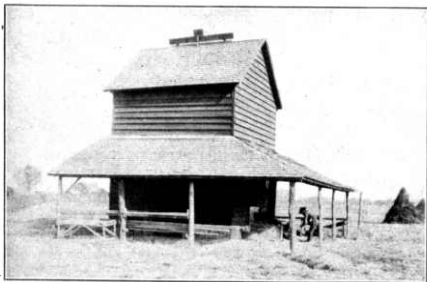
FIG. 1.—A 16 by 16 foot tobacco barn at the Pee Dee Experiment Station, Florence, S. C., which with slight modification served during the season of 1919-20 for curing tobacco from July 15 to September 1 and for sweet-potato storage from November 7 to March 25.
