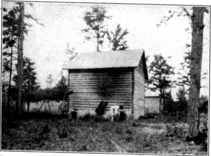
FIG. 3.—A typical log tobacco barn, showing the operator in the act of replenishing his fires.
