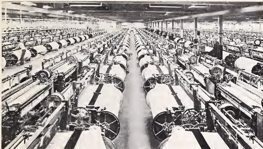
*Figure 23 Weaving—The loom is used for weaving yarn into fabrics by interlacing two systems of threads at essentially right angles to each other. The lengthwise threads are called warp yarn and the crosswise ones are the filler or “weft” yarn.*
