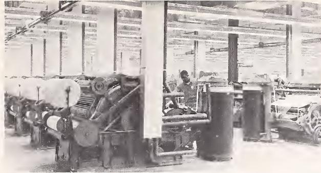
*Figure 17 Carding—After the picking process comes carding, which completes the cleaning action, removes short fibers, provides the first step toward bringing the fibers in a parallel order and produces a thin filmy sheet or web which is condensed into a rope-like, but untwisted strand about the size of a broomstick, known as a sliver.*
