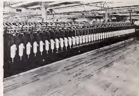
*Figure 19 Roving—The roving process which follows drawing is designed to reduce the cotton strand to a progressively smaller diameter, give it a slight twist, and wind it onto bobbins.*
