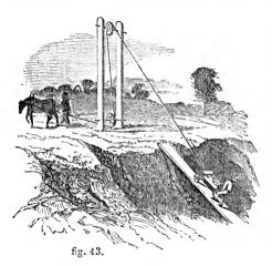
A curious illustration of the inclined plane and pulley was shown at the excavations of the Southampton and Sunderland Docks. A steep incline of planks, fig. 43, was laid down to the deep hole below, and a man hooking a rope on to a full barrow, which rope, passing over and under fixed pullevs, was attached to a horse, the animal received a stroke of a whip, walked sharply on, and the barrow, with the man taking long quick steps, leaning far out
