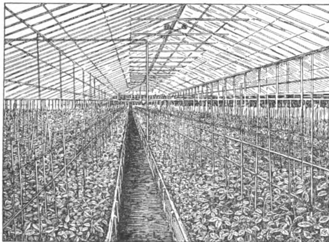
3482. Commercial rose-house showing method of staking, wood-bench construction, and connecting houses.
