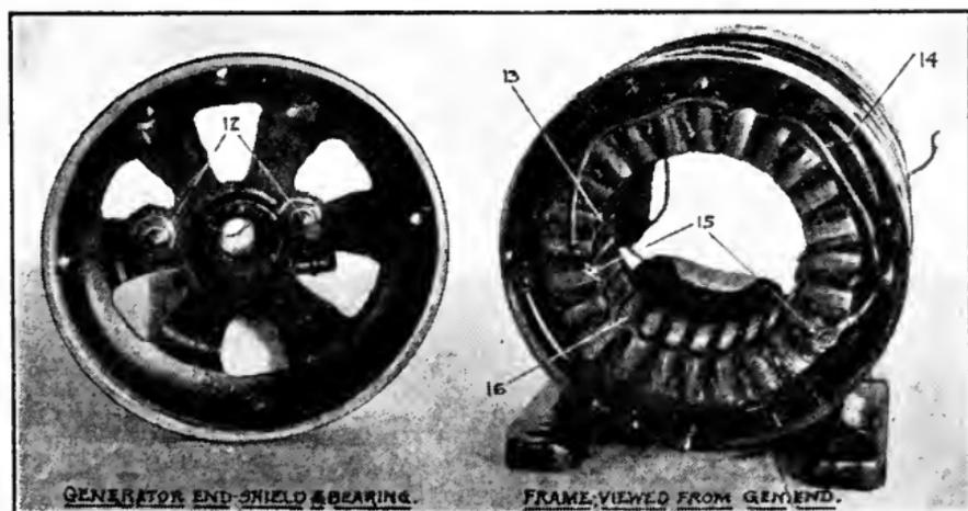
FIG. 122 (continued).—Motor-generator set of Fig. 121 partly dismantled.
