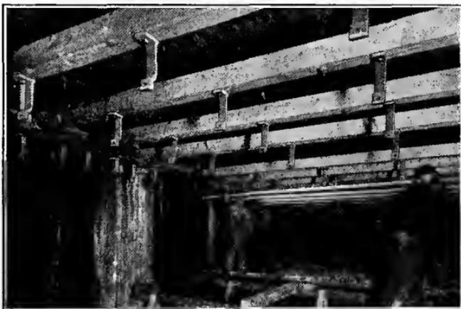
Showing insulation and meat rails being applied
