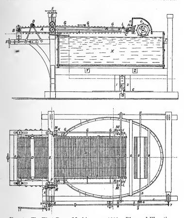
Fig. 4.—The First Paper Machine, A.D. 1802. Plan and Elevation. position on two rollers, one of which rotated freely in a bearing attached to the frame of the machine, the other being fitted in an adjustable bearing so that the wire could be tightened up when necessary.
