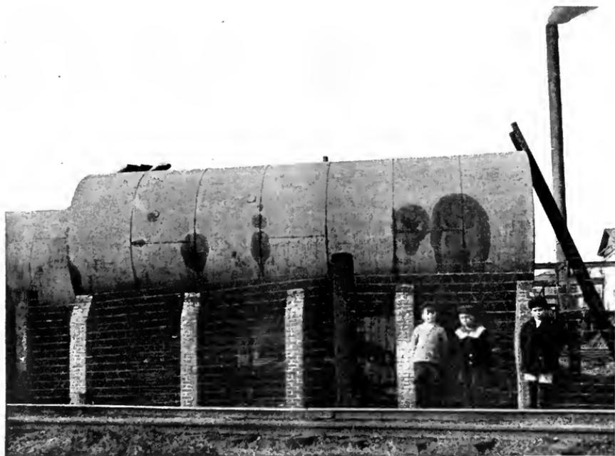
FIG. 2. THE PATCHED OIL TANK.
