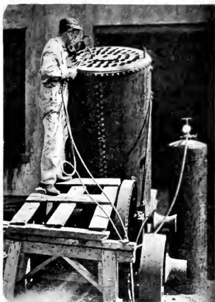
FIG. 1. WELDING TUBE SHEET.
