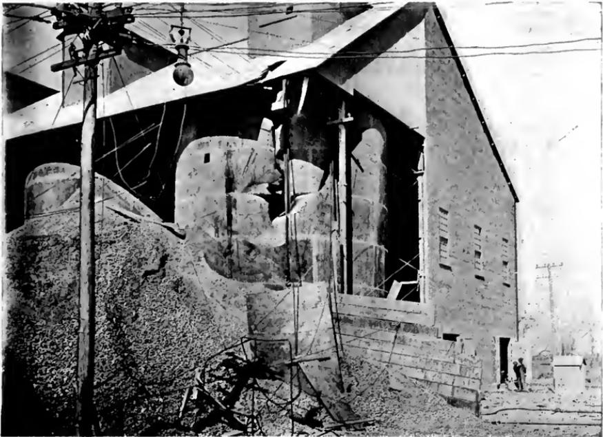
FIG. 6.—SHOWING THE DAMAGED STORAGE TANK.
