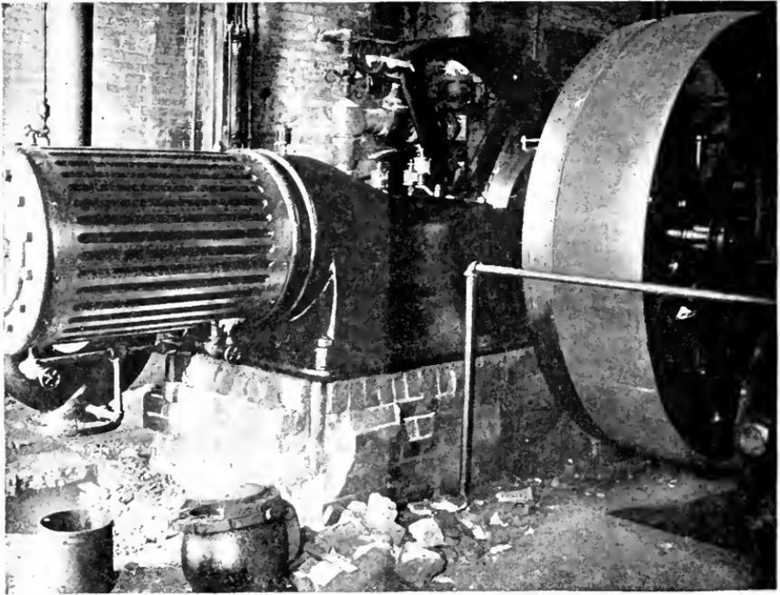
FIG. 5.— SHOWING THE DAMAGED FOUNDATION.
