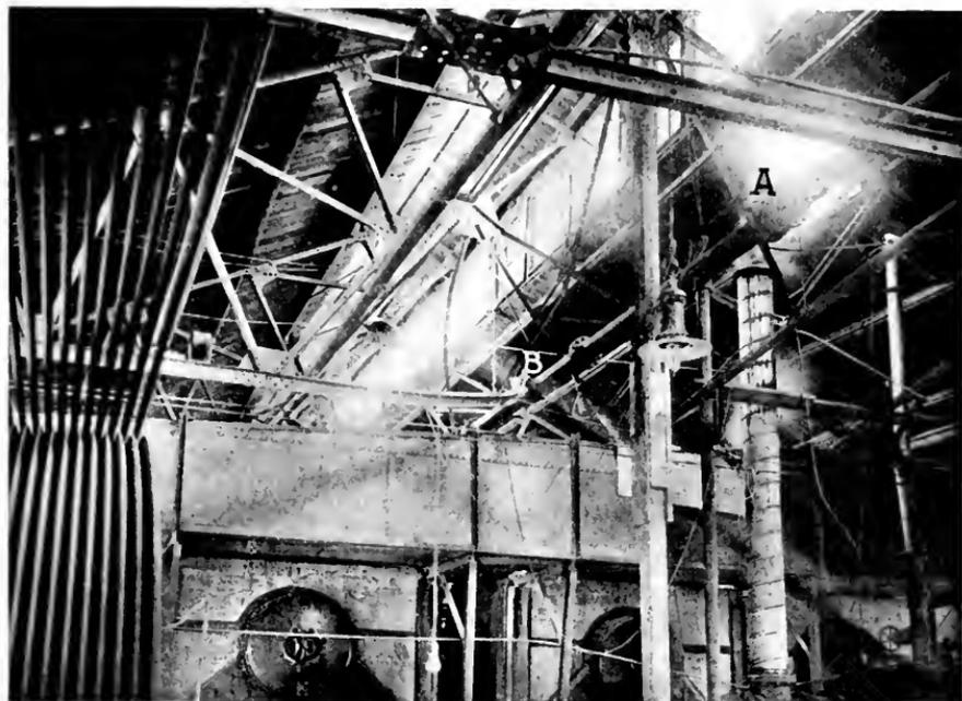
FIG. 5.— SHOWING THE EMERGENCY VALVE, A.
