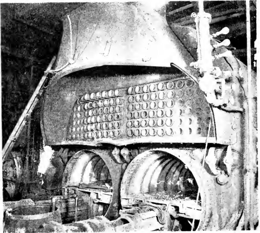
FIG. 1. DAMAGED FRONT OF BOILER.
