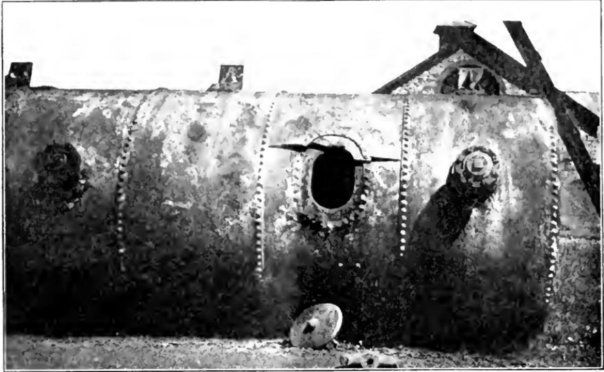
FIG. 2. SHOWING THE BLEEN MANHOLE FRAME OF BOILER 312.
