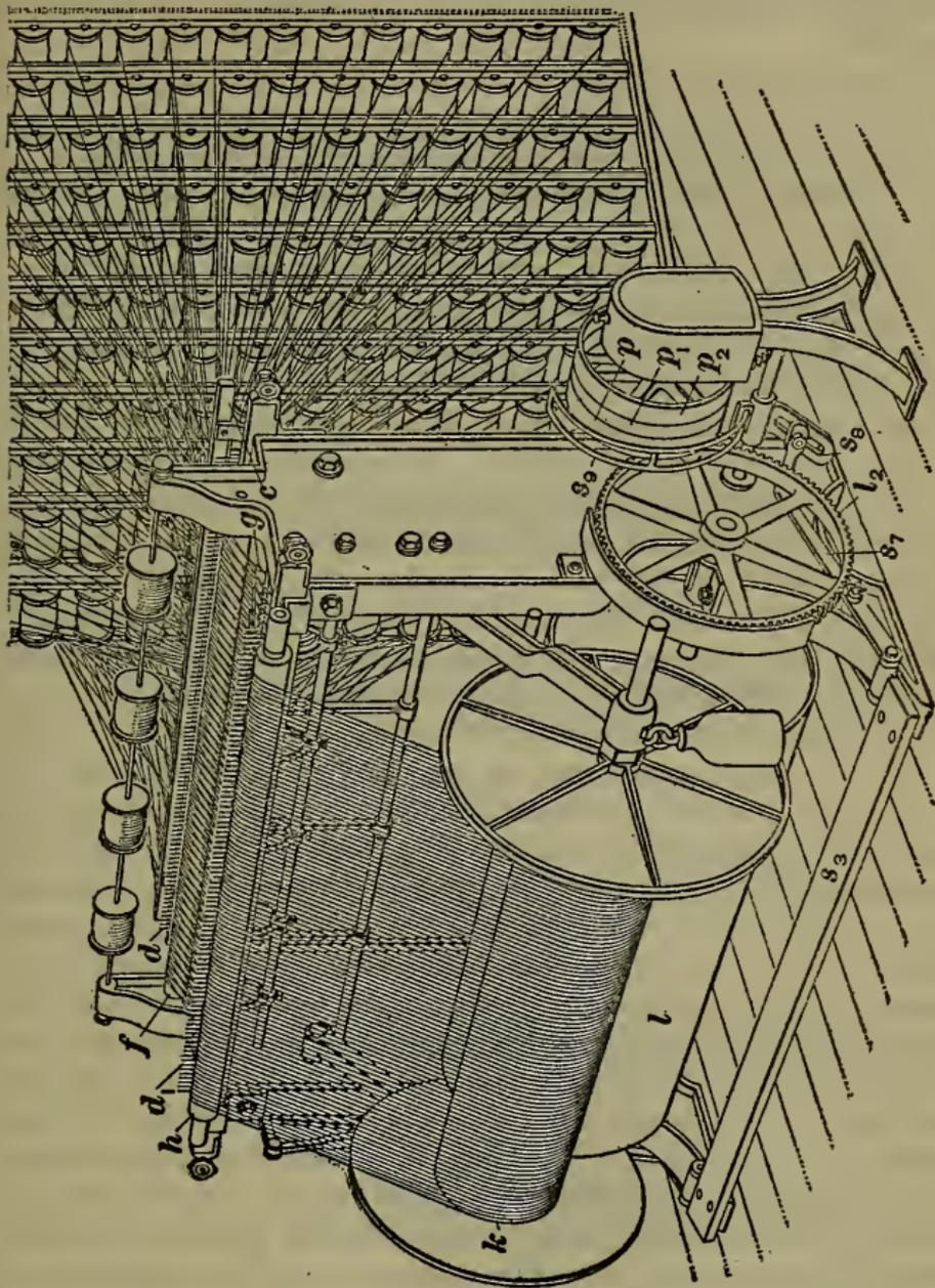
into contact with a drop roll, which takes up any slack yarn that may be let off by the spools, When the warper is stopped
