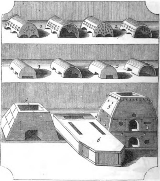
Fig. 137. "Nos. 1, 2, 3. Different forms of muffles. No. 4. An assay oven made of tiles joyned together, which may quickly be done. No. 5. An assay oven made of armour plate. No. 6. The foot of it." (Pettus.)
