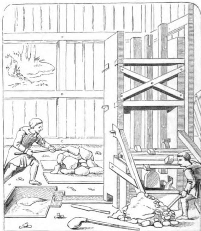
Fig. 163. Stampers and Box with Pits to receive the powdered Ore, used more than three hundred years ago. (Agricola.)
