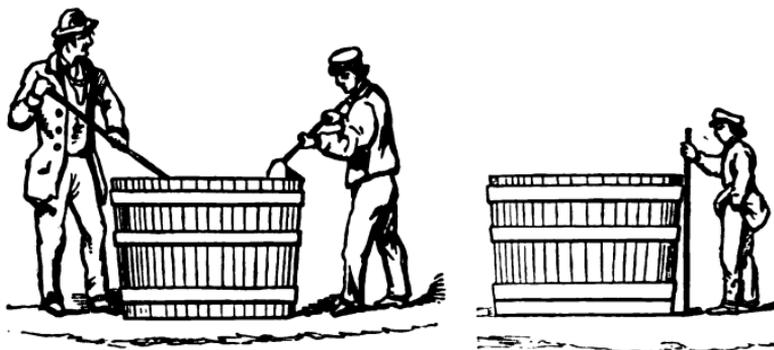
Fig. 177. Tossing and packing Tin Ores. (Henderson.)
