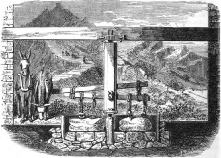
Fig. 132. A Crushing Mill used in Mexico.
