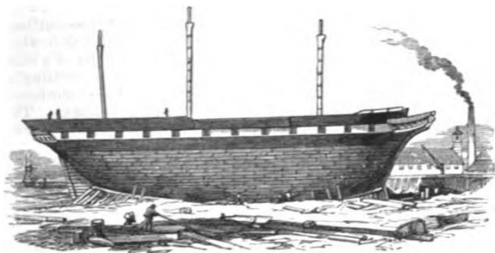
Fig. 173. Sheathing a Vessel with Copper.
