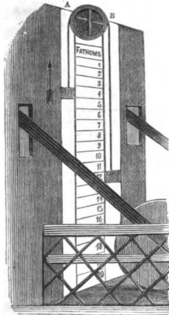
Fig. 39. The Tell-tale, which shows the position of the tube in the shaft.
