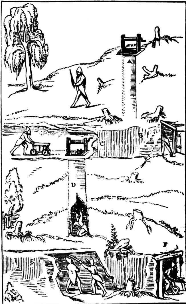
Fig. 10. A B. Main shaft. C B. Gallery heavily timbered. D. Shaft connecting the galleries with each other, called a winze. X F. Gallery timbered. (Agricola.)
