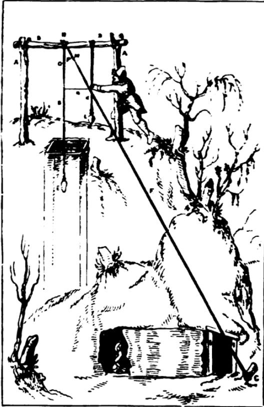
Fig. 147. The Adit Level. *a, a*. Two uprights or yokes supporting a bearer *b*. *c*. The well, pit, or shaft. *d*. First cord. *e*. Weight of the first cord. *f*. The second cord, fixed to the earth at *g*. *h*. Head or ends of cords. *i, i*. The mouth or entrance of the adit or tunnel. *k*. The third cord, with weight attached. *l, m*. The first measure; *n*, the second; *o*, the third, forming the triangle *p*. (Agricola.)
