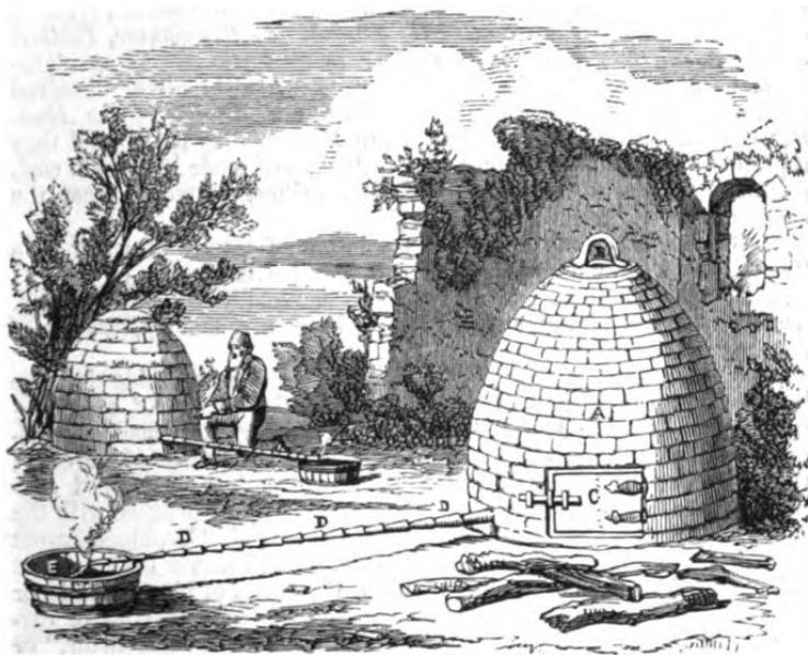
Fig. 91. Glauber's Method of procuring Acetic Acid by the destructive Distillation of Wood, copied from his "Miraculum Mundi." "A is the Furnace or oven, wherein the wood is char'd. B. The Cover of the Furnace. C. The door at which the coals are taken out D. The Canes or Pipes wherein the sap or juice of the wood is condensed, and from thence runs into the receiver. E is the vessell or receiver into which the vinegar of wood runs."
