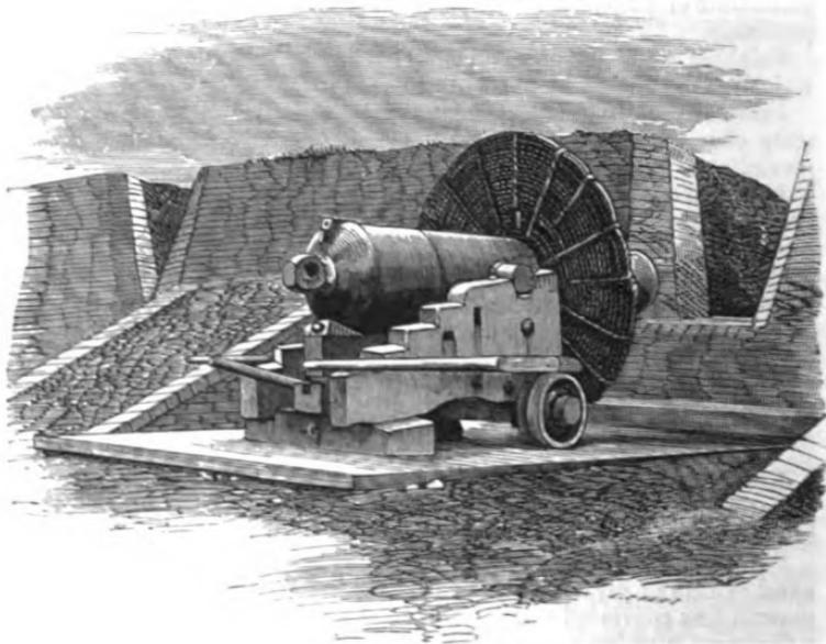
Fig. 219. Eight-inch Gun on Rear-chock Carriage, covered by the Russian Mantalet.
