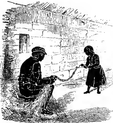
Fig. 529.— Making a straw-rope with a throw-crook.
