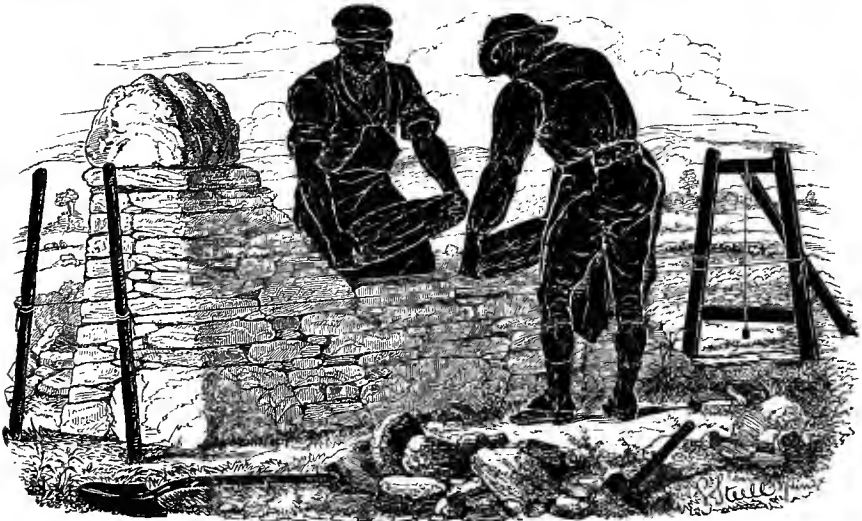
Fig. 574.—Building a dry-stone dyke.
