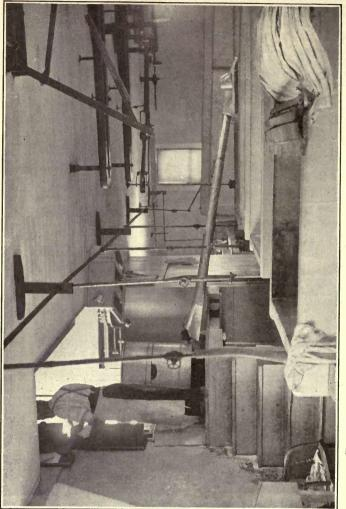
FIG. 30.— Receiving, sampling, weighing and running the milk into the cheese vat.
