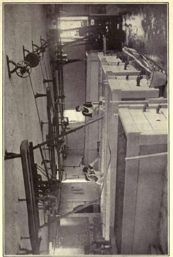
FIG. 35. - Two types of mechanical curd agitators.
