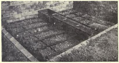
Tipping Apparatus and Distributor for Sewage Trickling Filter.
