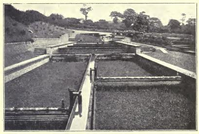
Fig. 20. Single-drum Travelling Distributor.
