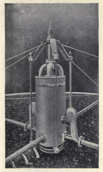
Fig. 45. Sprinkler with "Compensating" Arm.
