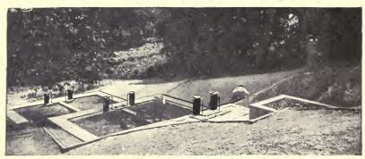
Automatic Alternating and Timed Discharge Syphons applied to Contact Filters.
