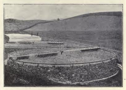
Fig. 19. Triple-drum Sprinkler on Circular Filter.
