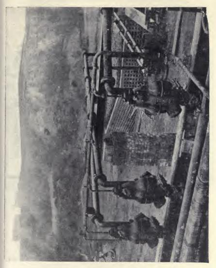
Fig. 38A. Application of Pulsometer Pump to Sprinklers.
