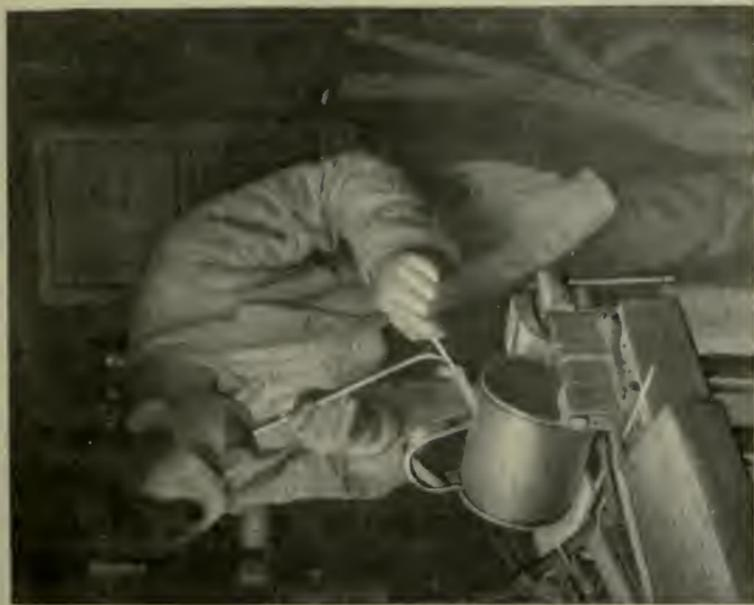
Fig. 35.—Soldering Lading-can handle
