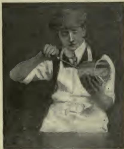
Fig. 20.—Soldering Internal Grooved Seam
