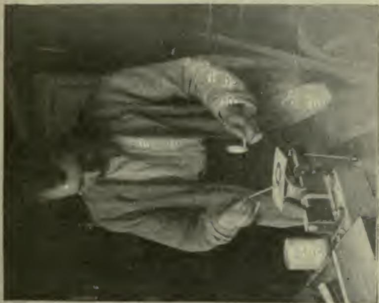
Fig. 39.—Brushing Solder around Dial Ring
