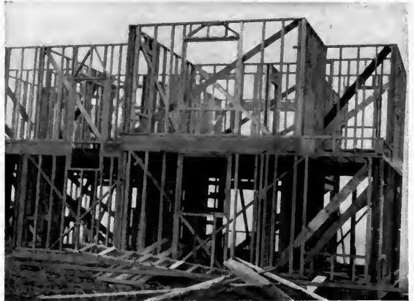
FIG. 109. A view from inside a frame house looking out. This shows the vertical two-by-four studs, the diagonal bracing between the latter, and the ceiling joists above.
