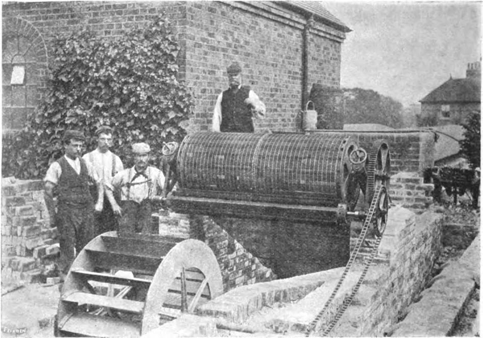
FIG. 17.—ROTARY SCREEN FOR CRUDE SEWAGE AT SOUTHALL SEWAGE WORKS, ISLEWORTH.
