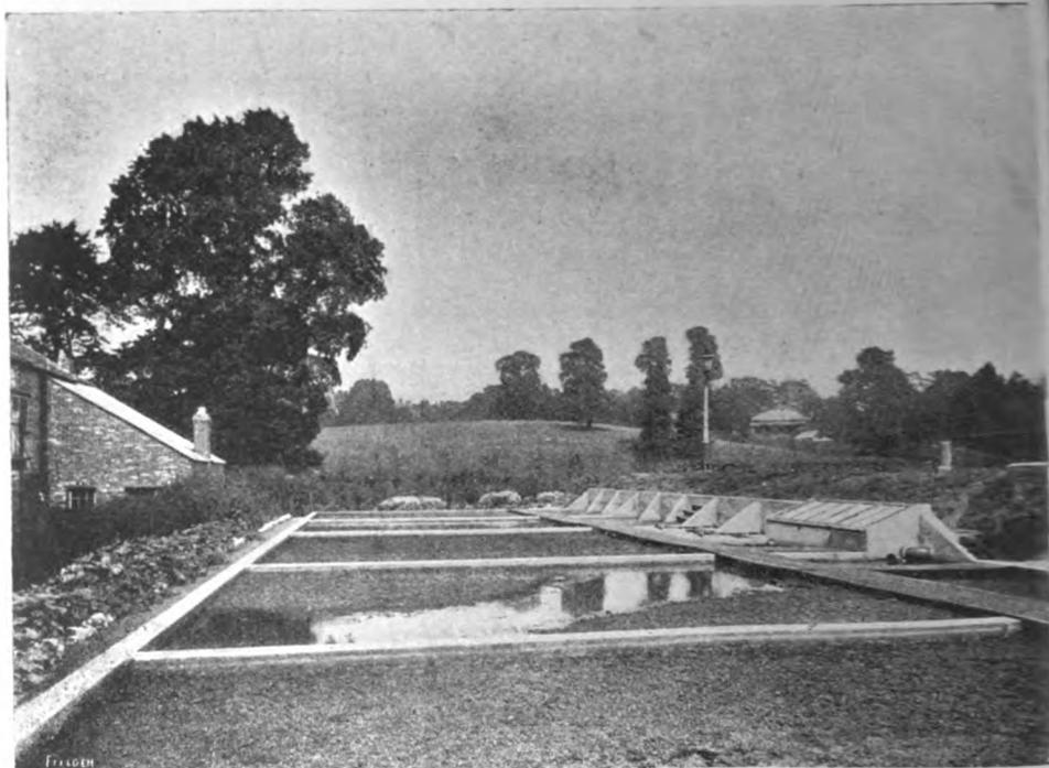
Fig. 33.—EXPERIMENTAL SEPTIC TANK AND FILTERS, BELLE ISLE, EXETER.
