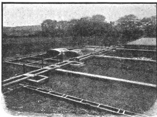
FIG. 23.—CONTACT, OR "DIBDIN" FILTERS ON DUAL SYSTEM AT SUTTON.
