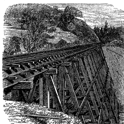
No. VI.—FIRST TRESTLE IN CLIPPER RAVINE.
