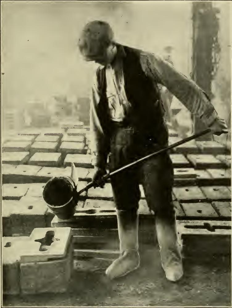
FIG. 4. POURING FROM A HAND LADLE.
