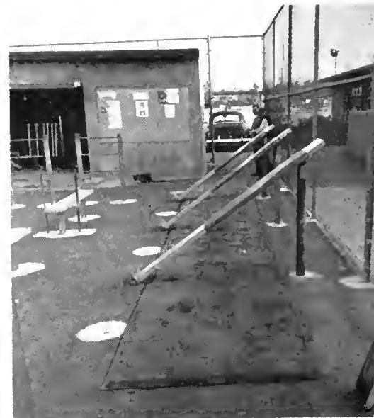
A weightlifting installation has a protective cushioning pad of Safety Surf. The maintenance costs have been nil.
