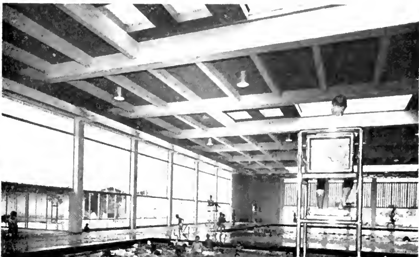
BUSY WATERS. Main pavilion of aquatorium shows training pool in foreground and Olympic pool in background. Sliding skylights admit bright California sunshine.
