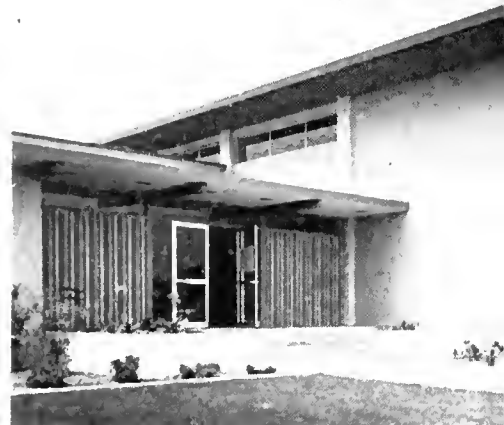
COMMERCE AQUATORIUM. Front elevation of huge re- at left, main pavilion enclosing two swimming pools, and
