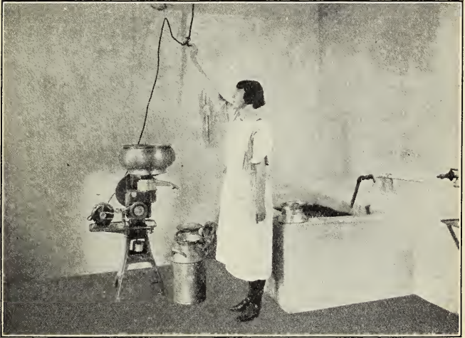
Cream at the turn of a switch. With electric transmission lines through country districts ever on the increase, farmers more and more are wiring their buildings for electricity. Electric operation of cream separators is easily accomplished; all the operator has to do is to connect the cord to any convenient lamp socket, turn on the switch, and let the motor do the work. The capacity of the electric cream separator shown in this picture is 75.5 gallons per hour.
