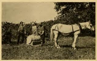
Fig. 189.—Barrel pump equipped for spraying in vineyard.
