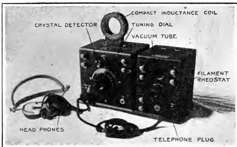
Receiving set making use of compact inductance coils for rapidly changing the wave length range in erg steps. The unit at right is the vacuum tube detector.
