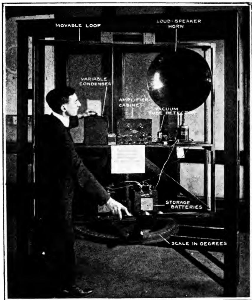
The radio compass which is employed as an aid in navigation. A number of turns of wire are wound about the large wooden frame which is rotatably mounted in the stationary frame, so that it can be orientated.
