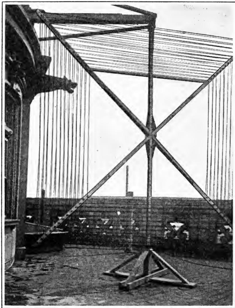
**Large loop antenna employed for the reception of trans-Atlantic messages by a New York newspaper. The loop is mounted so that it can be orientated or pointed towards the transmitting station.**
