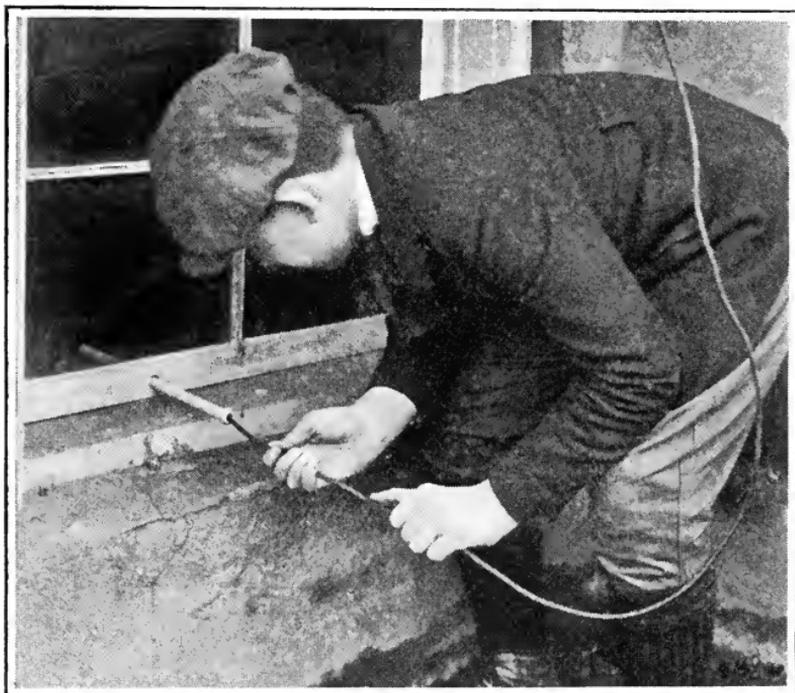
**It is best to pass all wires through porcelain tubes when they enter the house, as shown here, even though the wires may be heavily insulated. It is an additional precaution well worth taking.**
