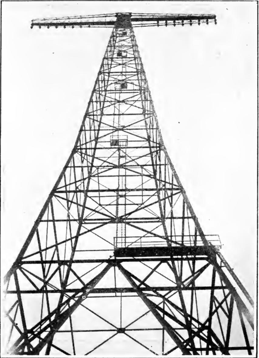
Looking up at the top of one of the steel towers of the Radio Central wireless station. The cross-arm at the top serves to support the sixteen wires which form the aerial.
