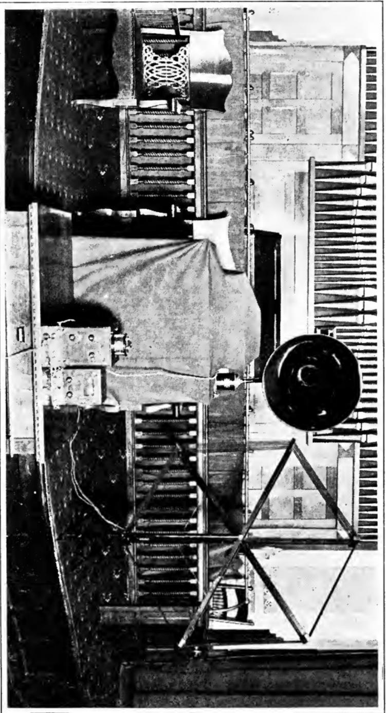
Radio receiving set installed in a Pittsburgh church in order to receive the church services and sermon from another church in the absence of the pastor. Note the loop antenna at the right, and the loud-speaker in the center.
