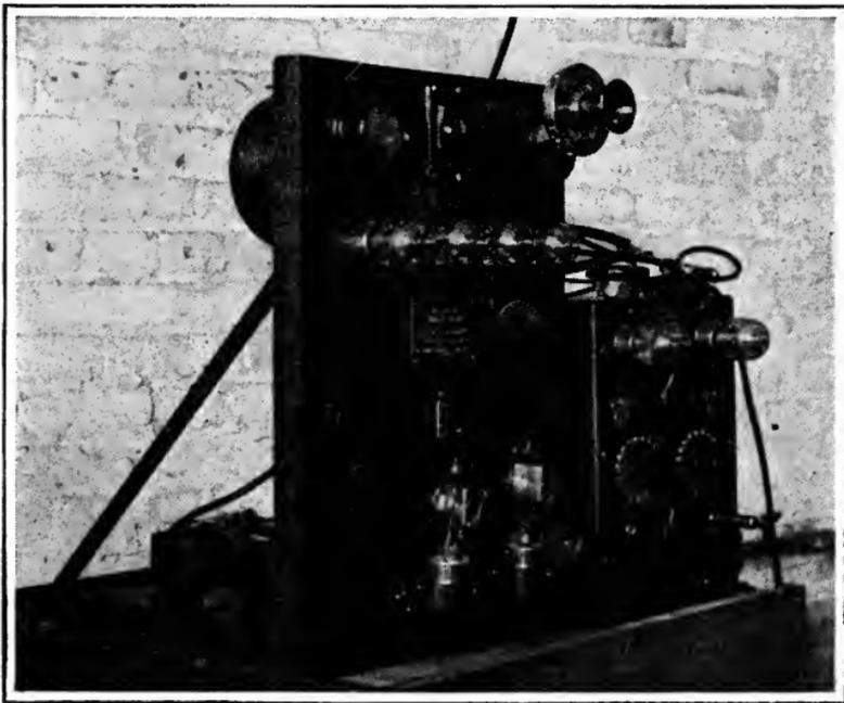
**Typical radio-telephone transmitter, which is provided with rectifying tubes so that it can be operated on an alternating current lighting circuit.**
