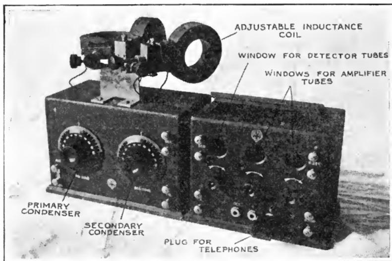
**Receiving set in which three compact inductance coils, adjustably mounted on top of cabinet, permit of variable coupling and regenerative action. The unit at right is the vacuum tube detector and two-stage amplifier.**
