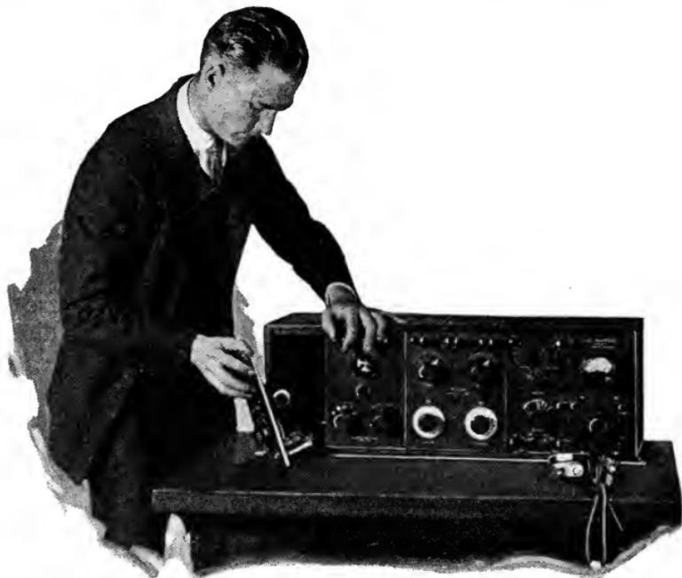
**The interchangeable panel idea is quite popular at present. Each component of a receiving set is mounted on a standardized panel, and as many panels as are desired can be used at one time with or without cabinets. The idea is quite similar to the sectional bookcase, which grows with one's needs.**
