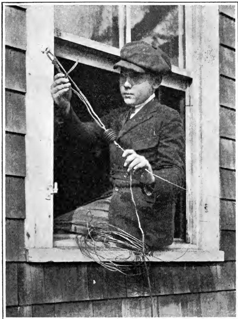
Nothing is simpler than erecting the antenna for receiving purposes. A single wire, with insulators at either end, is run between the house and a barn, tree, or clothes pole. Then a tap is taken off the near end of the antenna and brought into the house. This is known as the lead-in.
