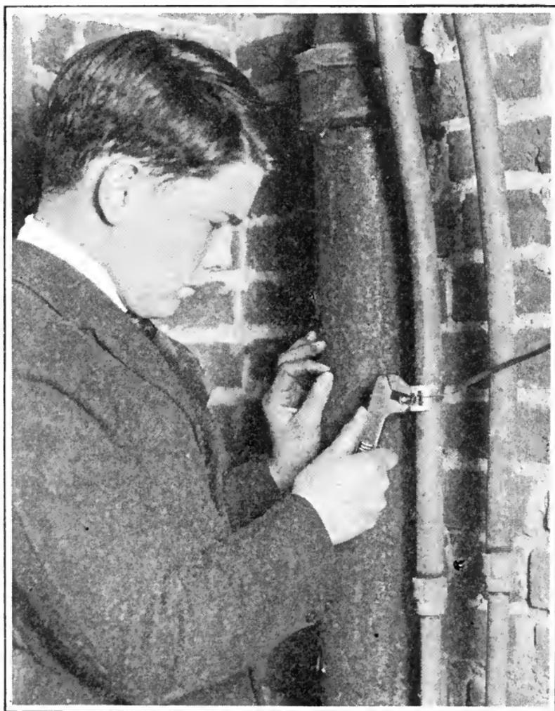
Too much pains cannot be taken with the ground connection. The ground may seem simple enough—and it is; but one should use a good ground clamp whenever possible, and connect it with the cold water pipe for best results, as shown here.
