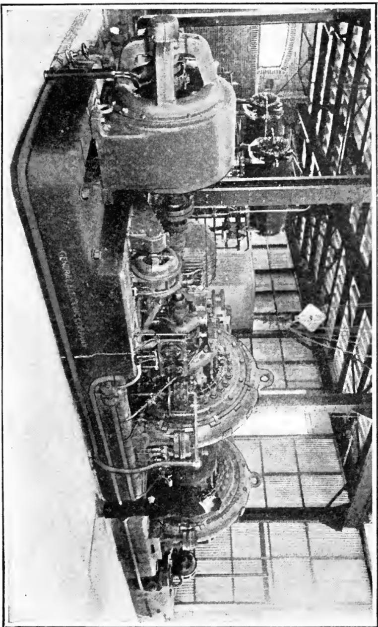
An Alexander-son 200-kilowatt high-frequency alternator as employed at the Radio Central wireless station and in other American long-distance stations. This machine generates high-frequency current and therefore takes the place of the usual spark oscillator.
