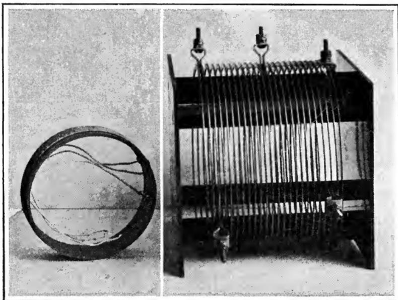
**Typical CW transmitting equipment, showing its simplicity. The coil at the left is a grid coil, while the instrument at the right is a transmitting helix, made up of a number of turns of flat copper strip. The clips are for the purpose of making the necessary connections at any points on the helix in order to obtain the proper wave length values.**
