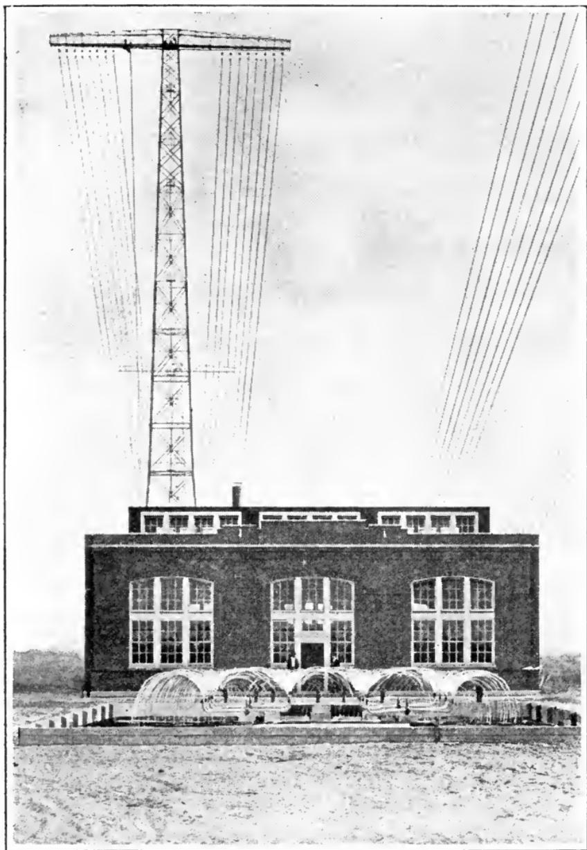
**The power plant and station building of the Radio Central wireless station. In the foreground are the sprays and cooling basin for cooling and condensing purposes, forming part of the power plant operation.**
