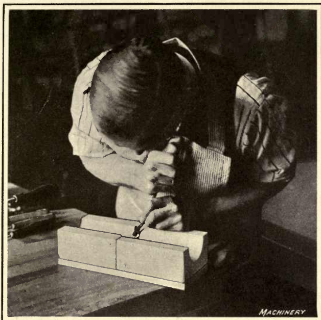
Fig. 10. Method of forming Fillet in Chambered Section of Core-box with Short-bend Carving Tool
