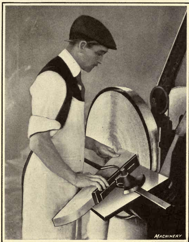
Fig. 15. Grinding End of Piece to a Double Angle on Disk Sander
