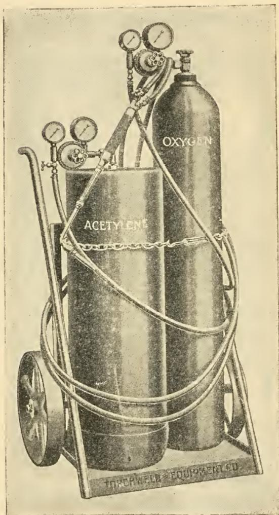
FIG. 14.—A Portable Welding Unit.
