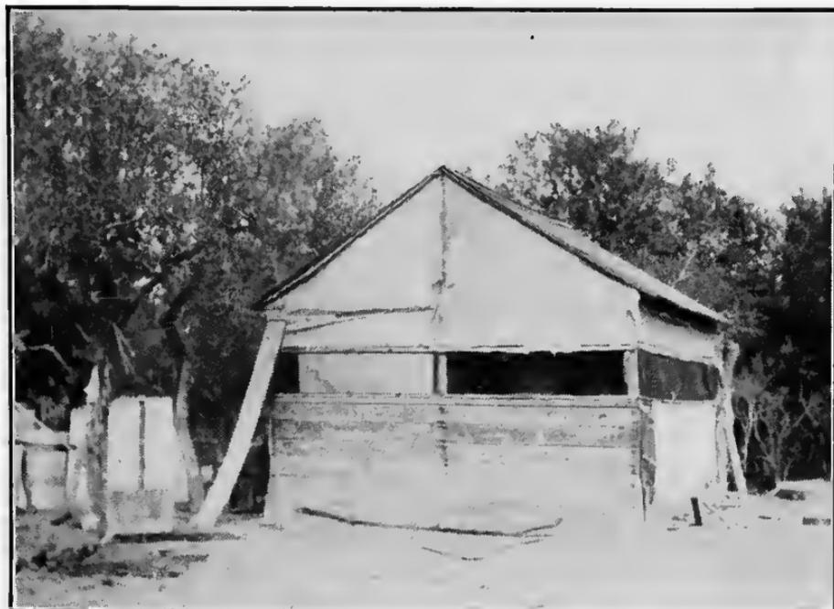
Fig. 55. Honey-house built with ample ventilation for extracting.
