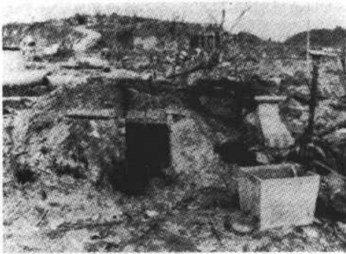
Fig. 1.5. Undamaged earth-covered family shelter in Nagasaki.
