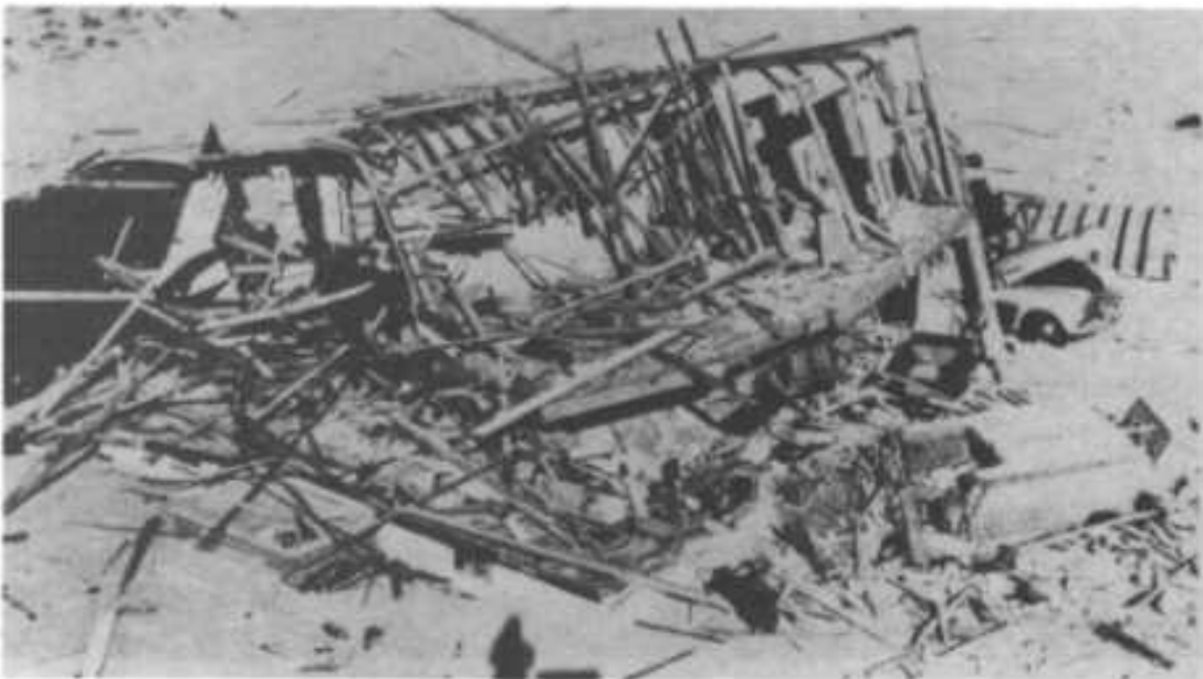
Fig. 7.4. Unburned wreckage of the same two-story, wood-frame house pictured in Fig. 7.1 after being wrecked by the 5-psi blast effects of a small nuclear test explosion.
