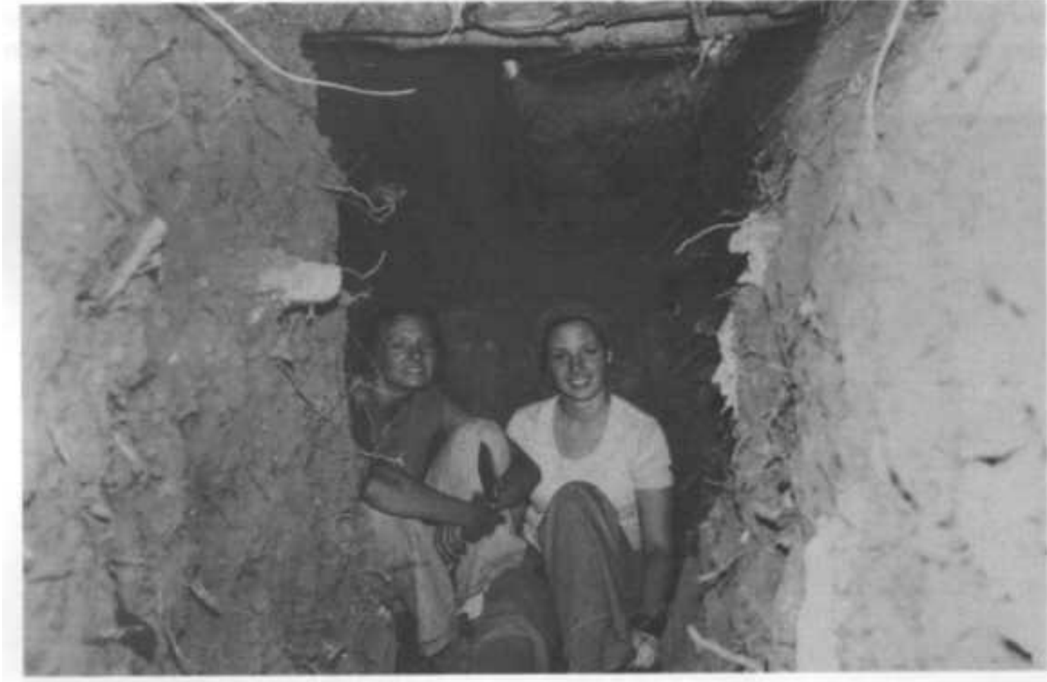
Fig. 5.2. Two non-athletic college girls who completed a 4-person Pole-Covered Trench Shelter in 35-1/2 hours, despite tree roots.
