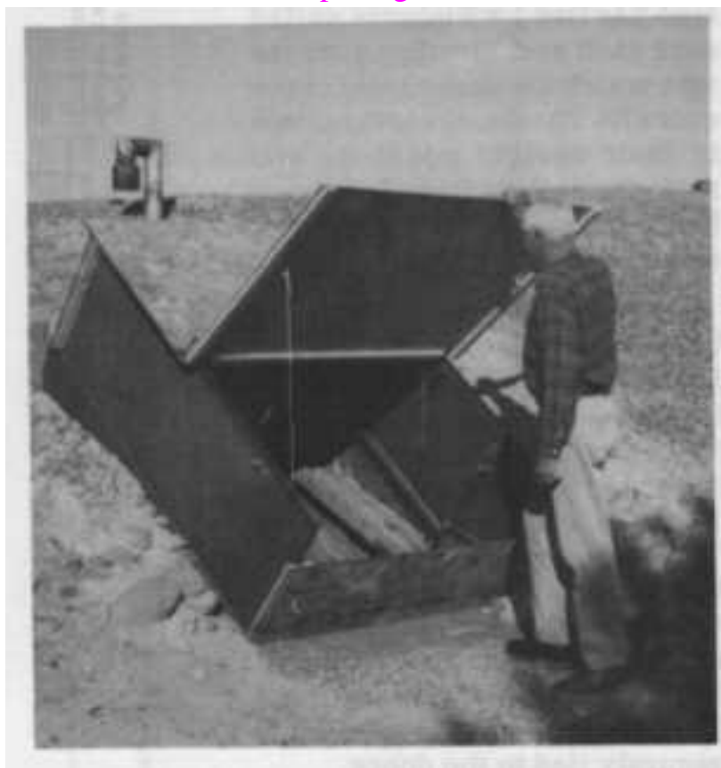
Fig. F.5. A Quickly Installable, 4-Piece Entryway Cover That Provides Easy Access and a Large, Protected Ventilation Opening.
