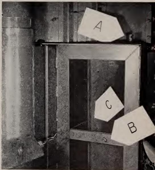
*Fig. 10.* A view of the back side of a pressure plate, showing (A) the spring tension adjustment; (B) the spindle clearance adjustment; and (C) the equipment for method of determining the yield pressure.
