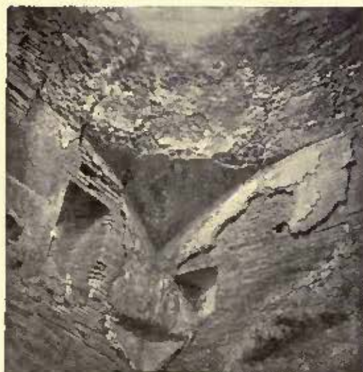
Fig. 47.—Rome. Tomb on the Via Nomentana. Pendentive of Dome (II nd Century).
