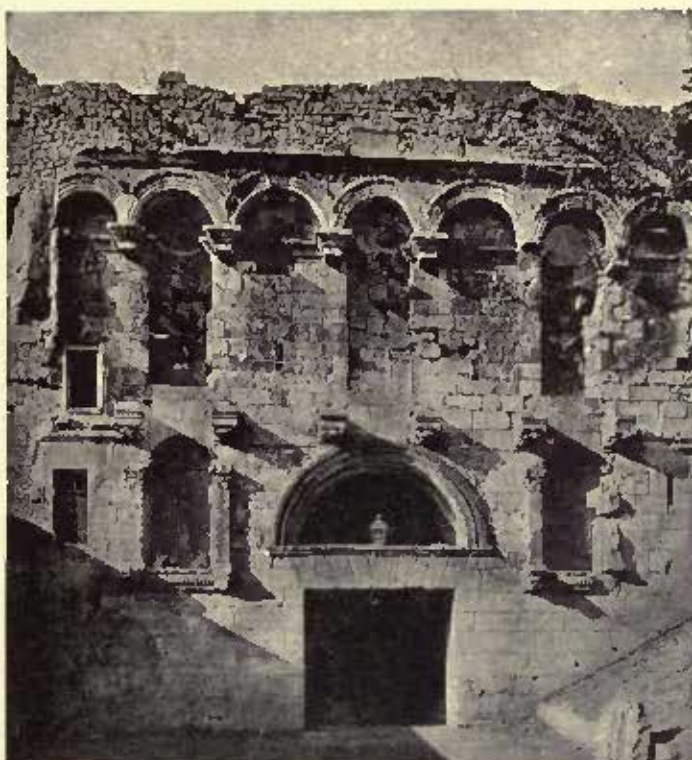
Fig. 144.—Spalato. Palace of Diocletian. Golden Gate (about 300-305).
