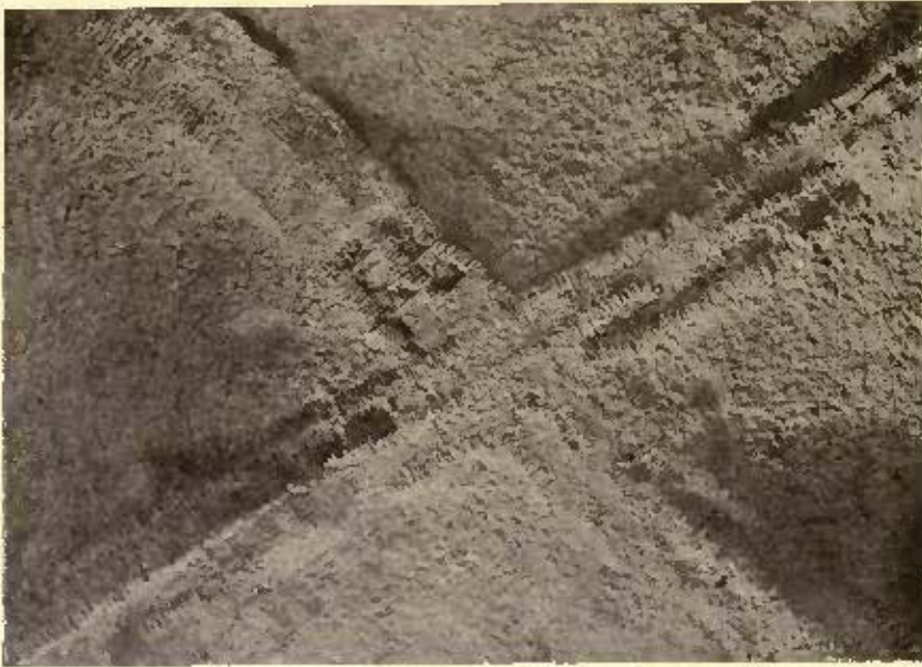
Fig. 123.—Rome. Baths of Diocletian. Ribbed Vault (306).
