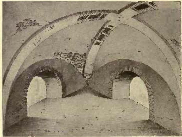
Fig. 361.—Rome. Villa called "Sette Bassi," Ribbed vaulting (12nd Century).
