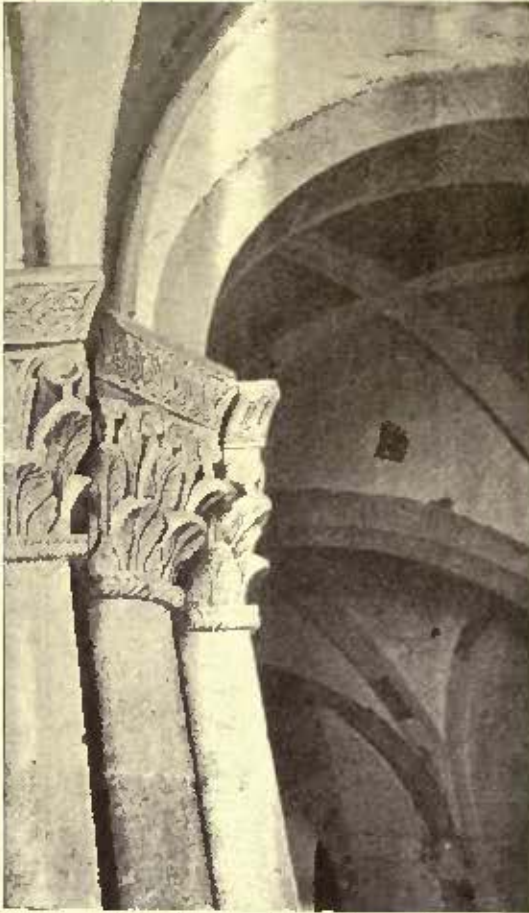
Fig. 303.—Montefiascone. San Flaviano. Vaulting of aisle (1032).
