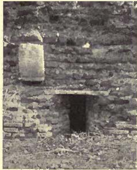
Fig. 140.—Rome. Villa called "Sette Bassi." Double-splayed window (100-155).
