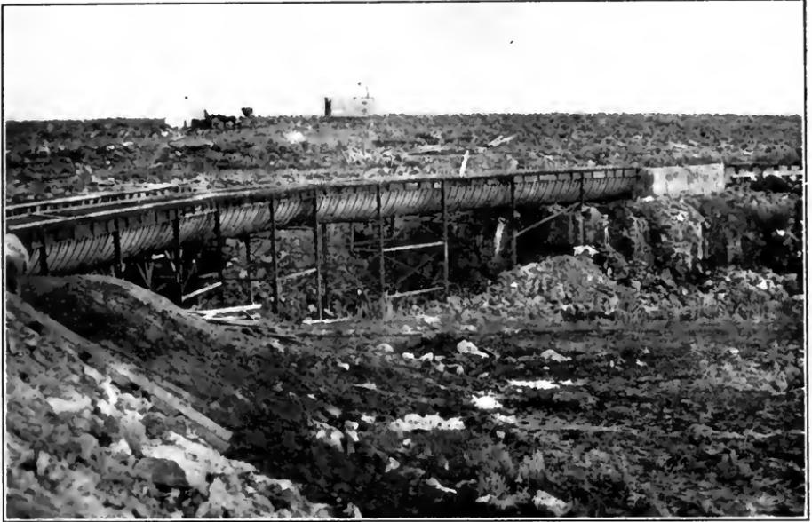
FIG. A.—Hess steel flume, 15 feet 6 inches diameter, on steel trestle. Twin Falls, North Side Irrigation Project, Idaho.
