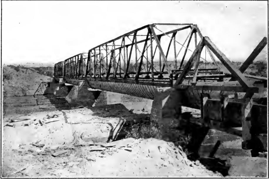
FIG. C.—Lennon steel flume, 6 feet 4 inches diameter, on 3 to 120-foot span steel bridge across Laptata River at Farmington, N. Mex., for Farmer's Mutual Ditch Co.
