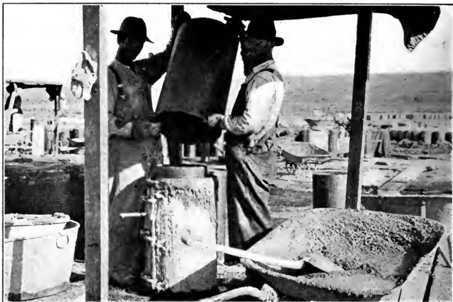
FIG. C.—Placing reinforcement cage, surrounded with tarred paper cylinder, in moulds. Tieton Project, Wash.
