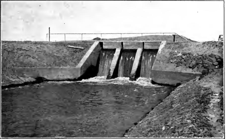
FIG. A.—Reinforced concrete drop. Truckee Carson Project, Nev.
