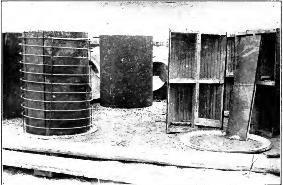
FIG. D.—Moulds for casting 30-inch reinforced concrete pipe. Umatilla Project, Ore.
