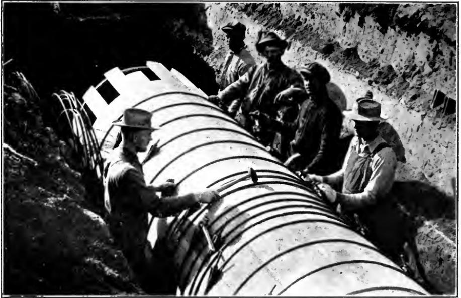
FIG. C.—Constructing a 45½-inch continuous wood stave pipe. Whittier, Calif.
