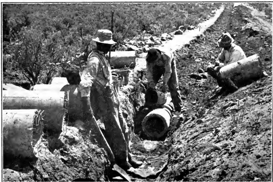
FIG. D.—Laying and joining reinforced concrete pipe. Tieton Project, Wash.
