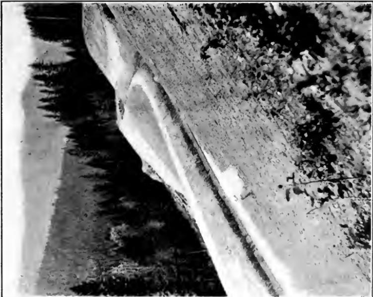
Fig. A.—Concrete-lined diversion canal on steep rocky hillside. South Kelowna System, B. C.
