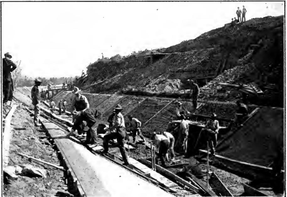
FIG. D.—Placing concrete lining. Ridenbaugh Canal, Idaho.
