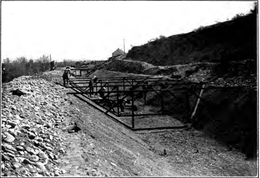
FIG. C.—Preparation of earth canal for concrete lining. Ridenbaugh Canal, Idaho.
