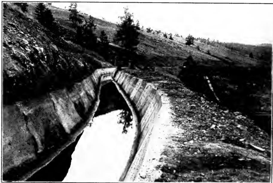
FIG. D.—Completed concrete-lined canal. Kamloops Fruitlands Irrigation & Power Co., B. C.
