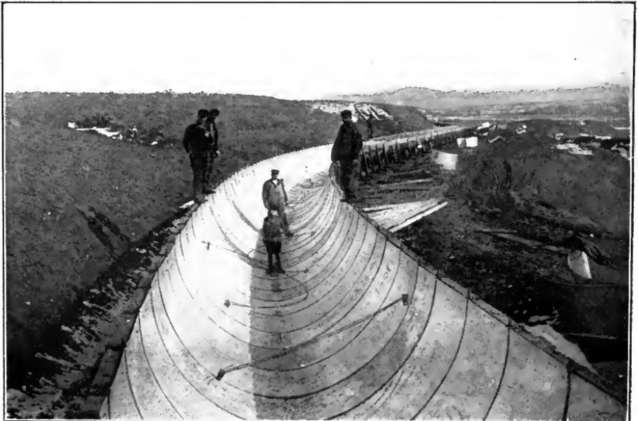
FIG. D.—Lennon steel flume—9 feet diameter. Trinchera Irrigation District, Blanca, Colo.
