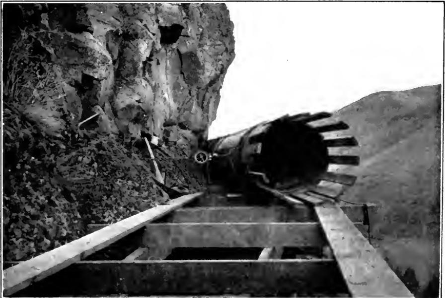
FIG. B.—48-inch wooden stave pipe (same as Fig. A) showing difficult construction of a curve on a steep bluff.
