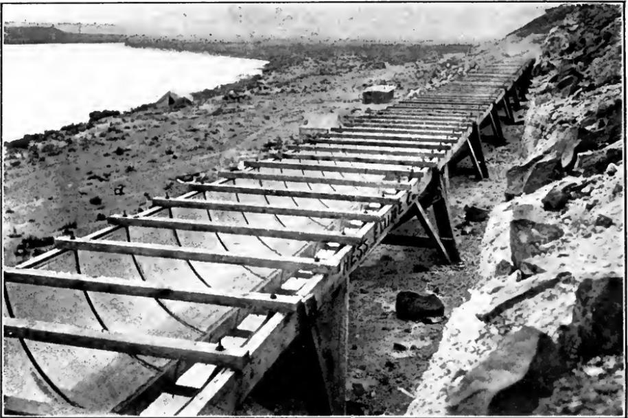
FIG. C.—Hess steel flume—7 feet diameter. Mountain Home Cooperative Irrigation Co., Idaho.
