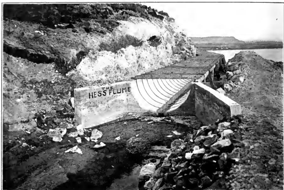
FIG. C.—Outlet to steel flume. Snake River Irrigation Co., Mountain Home, Idaho.
