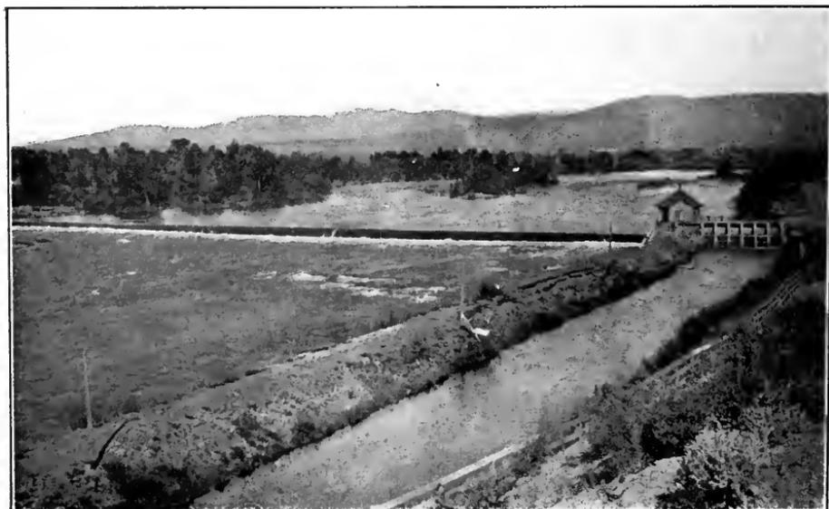
FIG. D.—Diversion weir and headworks of Sunnyside Project on Yakima River, Wash.
