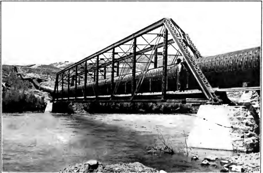
FIG. B.—60-inch continuous wooden stave pipe on bridge over Bear River, Oneida Irrigation District, Idaho. 300-foot head,  $\frac{3}{4}$ -inch bands,  $\frac{5}{8}$ -inch center to center. (Pacific Tank & Pipe Co.)
