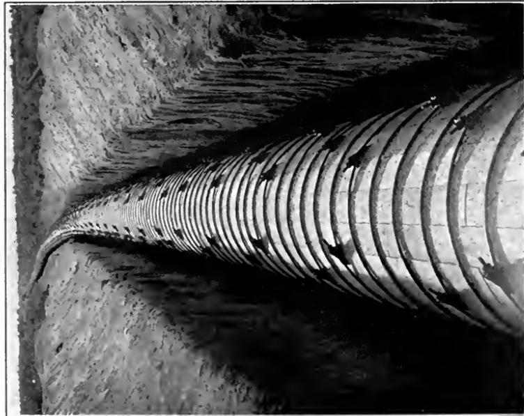
FIG. A.—36-inch continuous wooden stave pipe. Eastern Washington (Washington Pipe & Foundry Co.).
