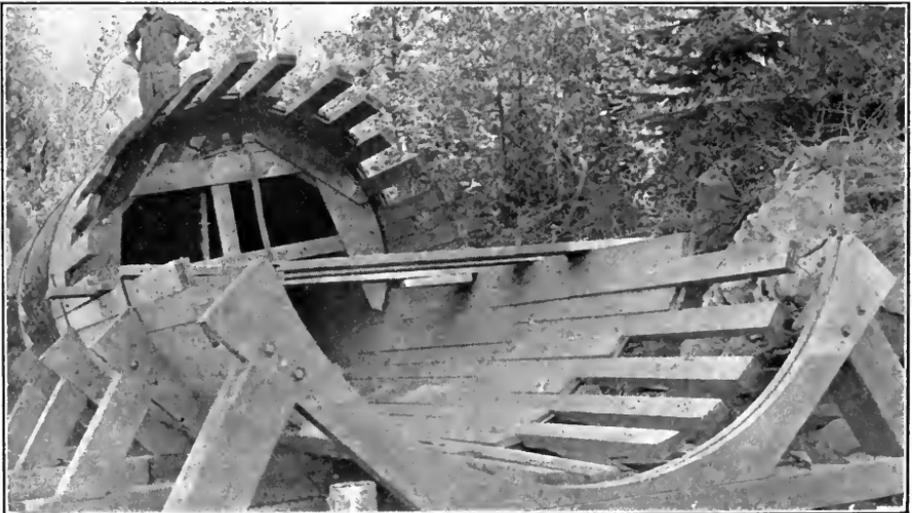
FIG. D.—Construction of wooden stave pipe on cradles.
