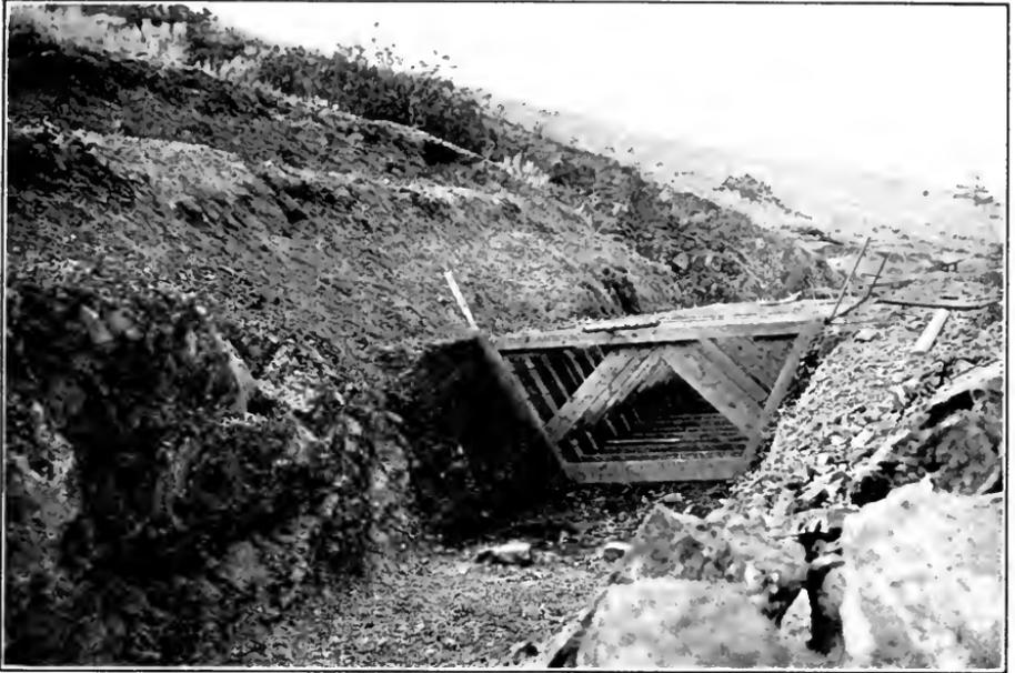
FIG. A.—Forms in place, to shape canal for concrete lining. Kamloops Fruitlands Irrigation & Power Co., B. C.
