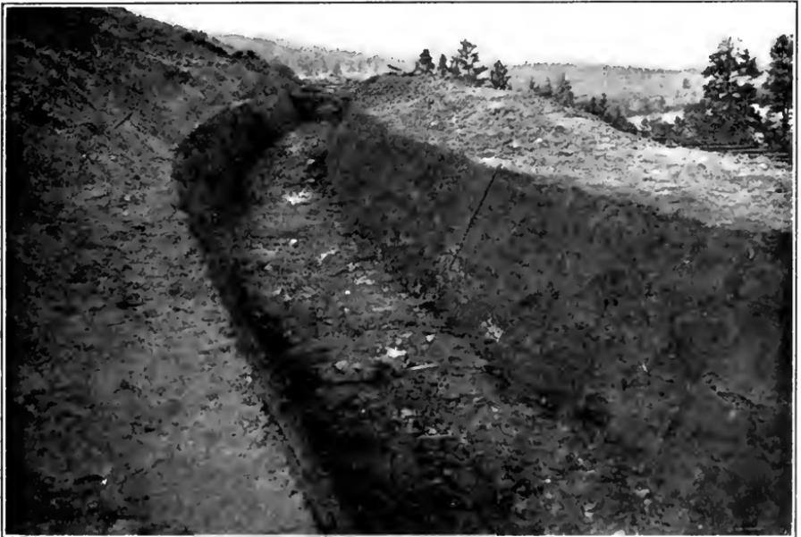
FIG. B.—Finished earth canal, ready for concrete lining. Kamloops Fruitlands Irrigation & Power Co., B. C.
