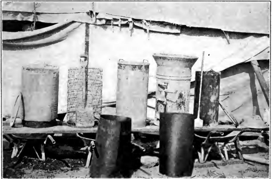
FIG. B.—Moulds for making small size reinforced concrete pipe. Tieton Project, Wash.
