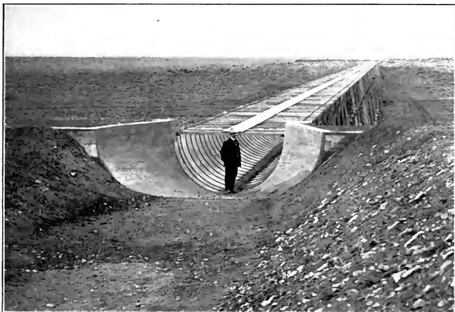
FIG. A.—Warped wing inlet. Twin Falls, Salmon River Land & Water Co., Idaho.
