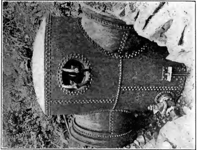
Fig. B.—Anchor well used at angles on 60-inch pipe line of Denver Union Water Co., Colo. (Eng. Rec. 18, 1912.)
