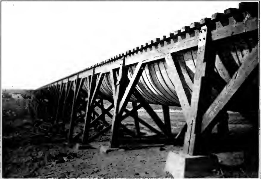
FIG. B.—Hess steel flume, 10 feet 10 inches diameter. Belle Fourche Project, S. D.
