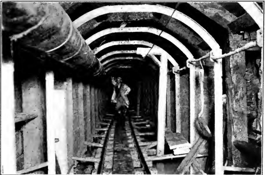
FIG. B.—Interior of Strawberry Valley Tunnel, in timbered section; steel ribs in place for supporting concrete forms; tramway and trolley; ventilation pipe. Strawberry Valley Project, Utah.
