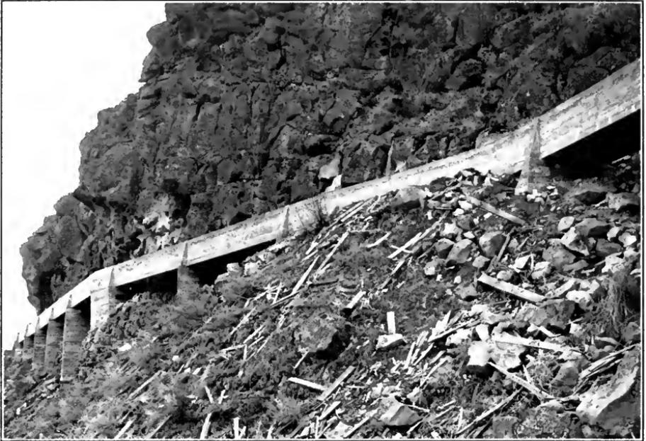
FIG. C.—Reinforced concrete flume. Naches Power Co., Wash.
