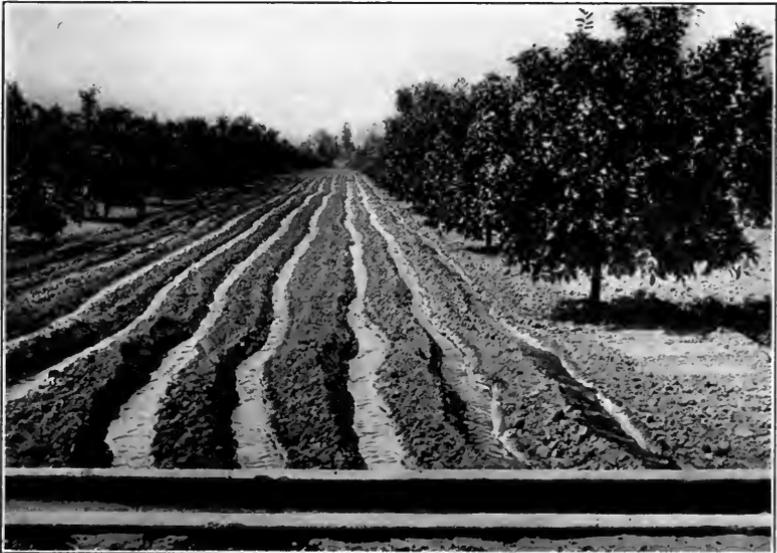
FIG. B.—Furrow irrigation from concrete head flume.
