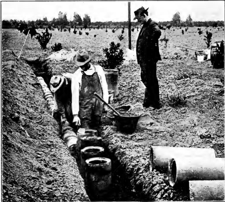
FIG. D.—Laying concrete pipe.
