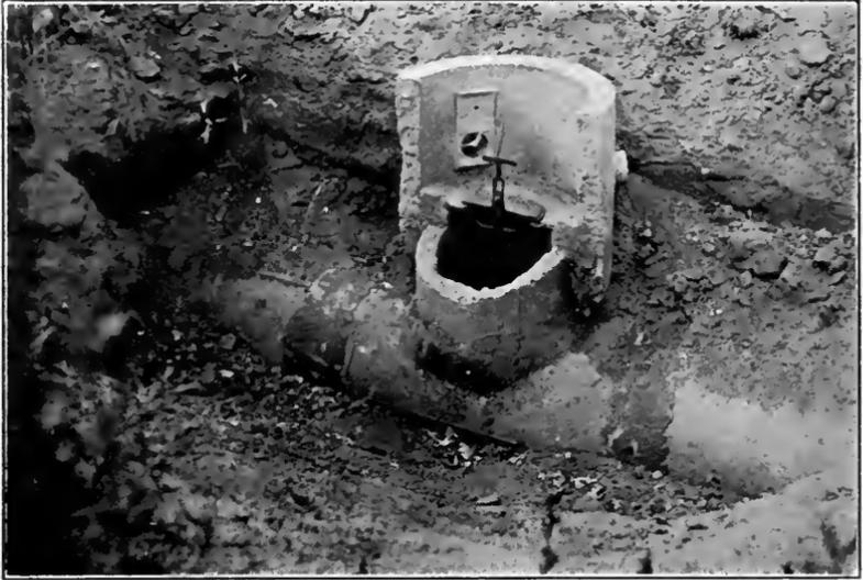
FIG. C.—Distributing pressure stand pipe, with valve.
