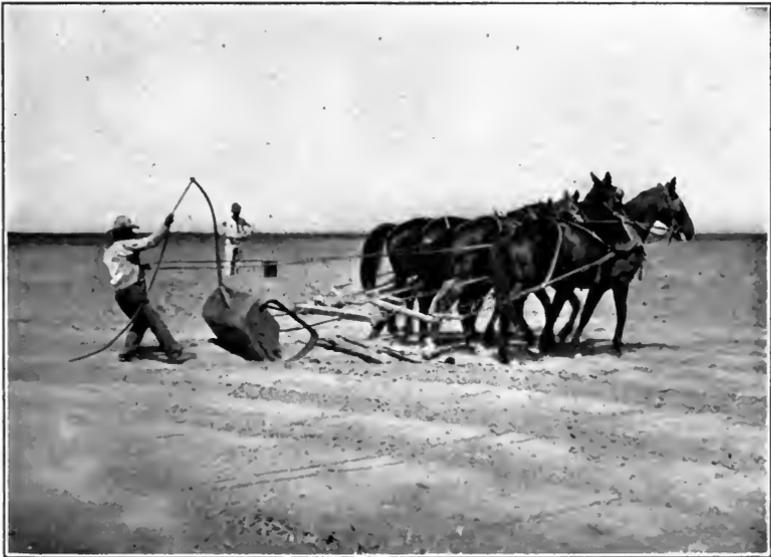
FIG. B.—Levelling the land surface with Fresno scraper.
