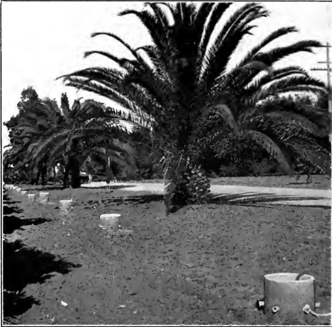
FIG. C.—Line of distributing stand pipes for distribution of water from cement pipe.
