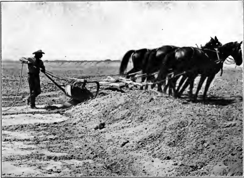
FIG. A.—Constructing levee for check method of flooding, with Fresno scraper.
