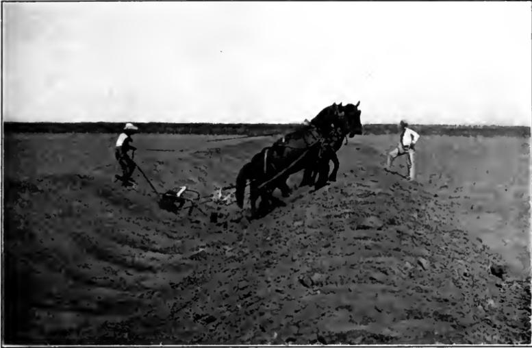
FIG. A.—Constructing farm ditch with Fresno scraper, near Modesto, Calif.
