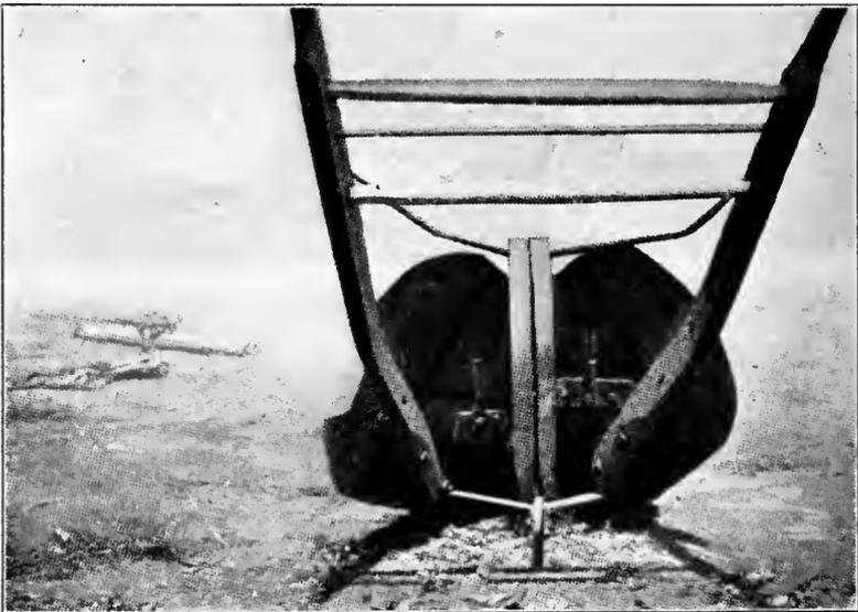
FIG. D.—Plow for making field ditches, made of right and left plows.
