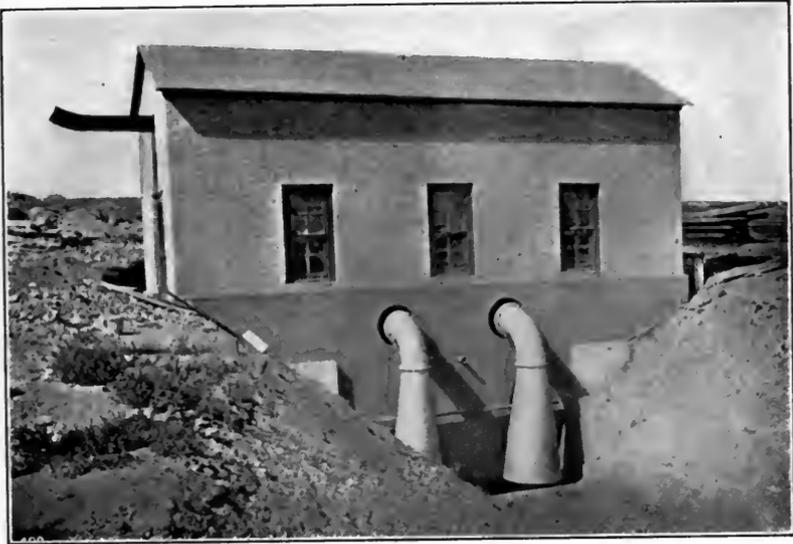
FIG. A.—Pumping plant installation for water supply obtained from an irrigation canal.
