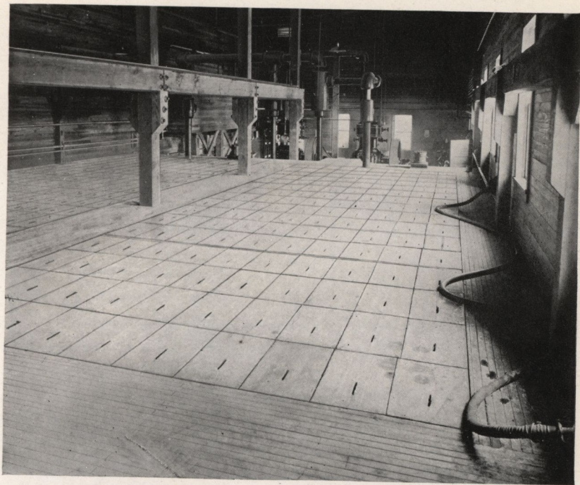
Freezing Tanks—Raw Water System
