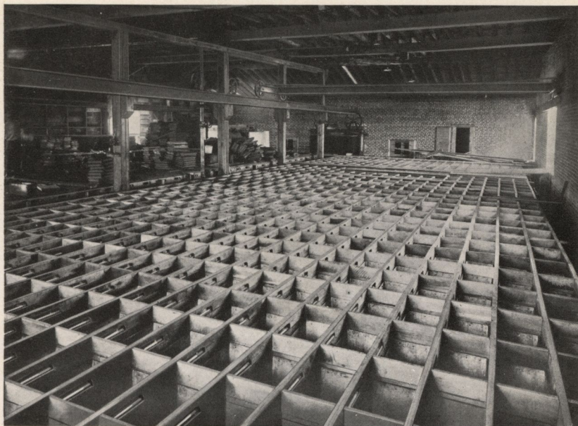
Freezing Tank Framework
