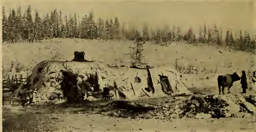
Fig. 44. A Yakut Dwelling. A double structure is shown, a dwelling with chimney, and a cattle stable, adjoining. Inside the dwelling a door leads to the stable. New-born calves are kept in the dwelling behind the chimney.
