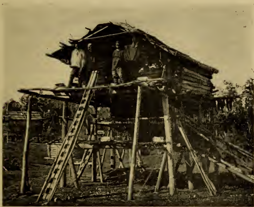
Fig. 52. A Kamechadal Storehouse which also serves as a Summer Dwelling. Such houses have two or three floors and in the upper one food is stored out of reach of the dogs. The lower floors are used for storing clothes and household belongings.
