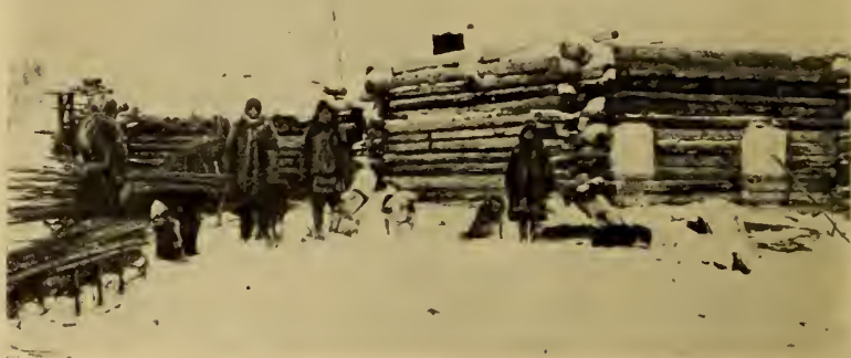
Fig. 45. A Flat-Roofed Blockhouse of the Upper Kolyma Yukaghir which serves as a Winter Dwelling. The windows are covered with thick panes of river ice.
