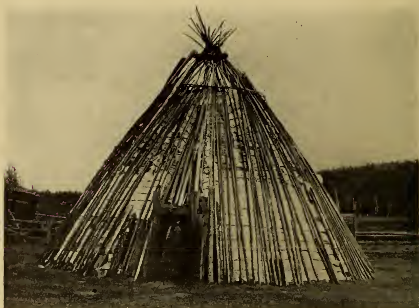
Fig. 33. Summer Dwelling of the Ancient Yakut. These were large conical tents, covered with birchbark, often elaborately decorated, but now seldom seen.
