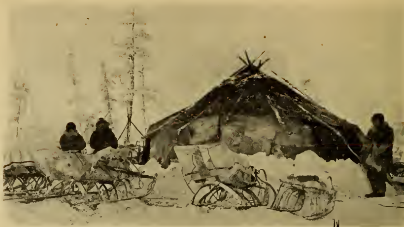
Fig. 38. A Cylindro-Conical Tent of the Tundra Yukaghir. It is covered with reindeer skins; in the winter, with the hair on; in summer, without the hair. In winter the lower part of the tent is banked with snow for warmth. The photograph is from the rear, where covered freight sledges serve as storage places for clothing and household belongings.
