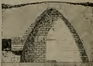
FIG. 6.—SECTION OF THE TREASURY OF ATREUS AT MYCENÆ.
