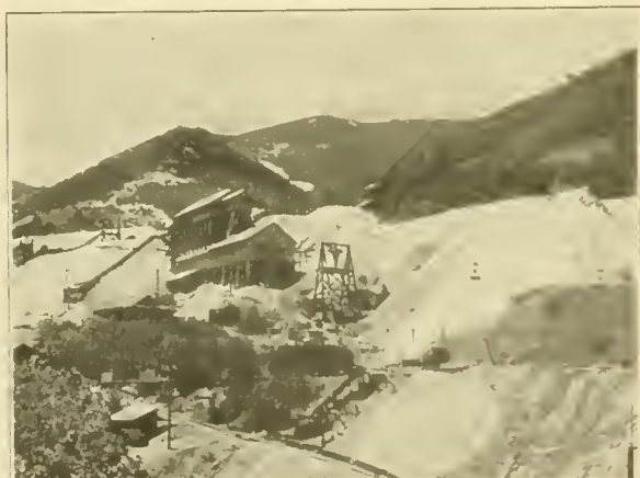
FIG. 41. Head house, Galena mine, Bingham Canyon. Notice the aerial tramway for sending the ore below.
