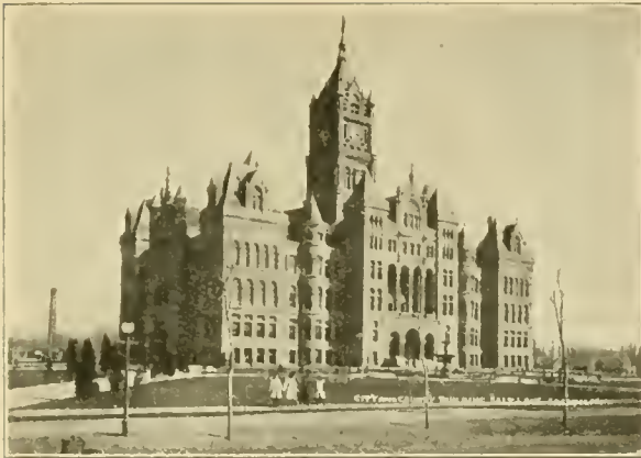
FIG. 63. The City and County building, Salt Lake City.
