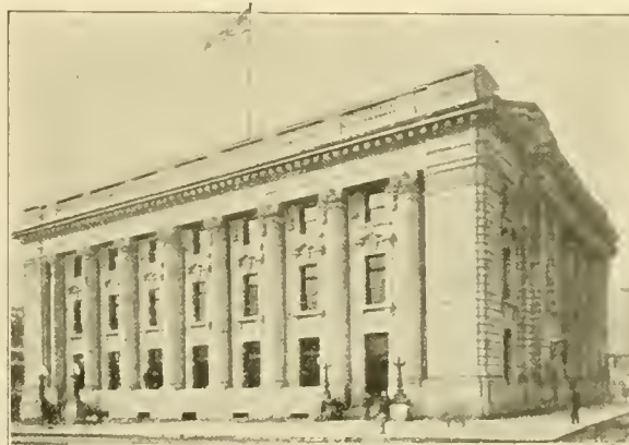
FIG. 53. The Federal Building, Salt Lake City.
