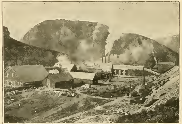
FIG. 45. A sampling mine in Bingham Canyon. Here the ore is concentrated, or separated from the rock, and only the richest shipped to the smelter.
