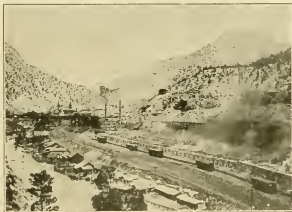
FIG. 40. Coal mines and coke ovens, Castlegate. Coal from this field produces coke which, as an ideal fuel for industrial plants, bids fair to rival the celebrated Connellsville product.
