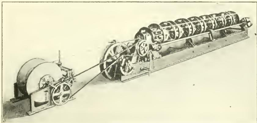
FIG. 36. A machine which twists the wires into strands
