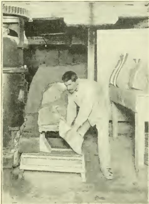
FIG. 50. This man has in his hands a block of clay which is ready to be pressed and molded
